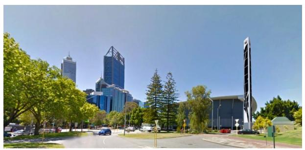
The Mosaic structure is modular, comprising an integral equipment room at the base and a number of tower sections. The antennas are mounted on the top sections. Mosaictower is available for site sharing of up to three carriers and with heights up to 36m.
