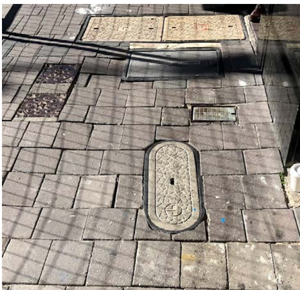
Figure 4: Typical Hobart CBD footpaths which were built in perfect condition but have sunk, cracked, been left with trip hazards and been artificially degraded by multiple carriers (and others) competing for limited space. Carriers and their contractors take no responsibility for these works as poor engineering is usually not revealed until later when they can claim subsequent events have degraded their installation. Often, no single installer/contractor can successfully be pursued for poor engineering practices since each will blame issues on other contractors. We do not have the resources to pursue every instance or take these issues to court, so ratepayers are left to repair streets and essentially subsidise poor quality work. The overall effect is an ugly, unsafe surface and a poorly-designed space. 5G will see orders of magnitude more requirement for CBD infrastructure in already overcrowded sub-surface space.
