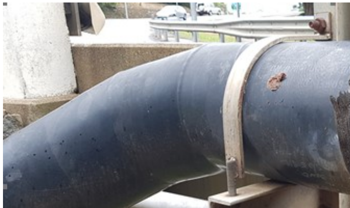
Figure 1: Telecommunications conduit installed through a water pipeline bracket attached to a bridge.
