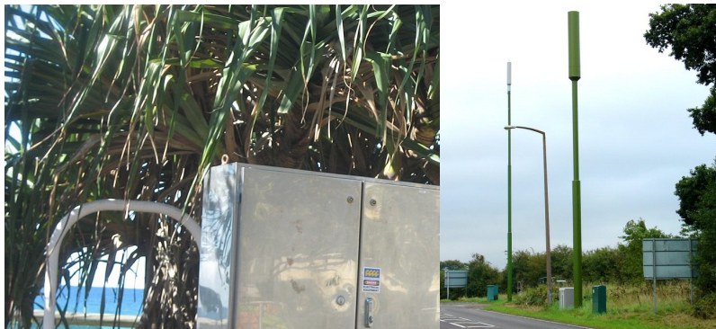
Figure 8: Example of what an aboveground cabinet for a small-cell split installation is expected to look like in a road. Dimensions for a small cell cabinet are expected to be approximately 1300mm high x 800mm long x 520mm wide. (Images © Creative Commons)
