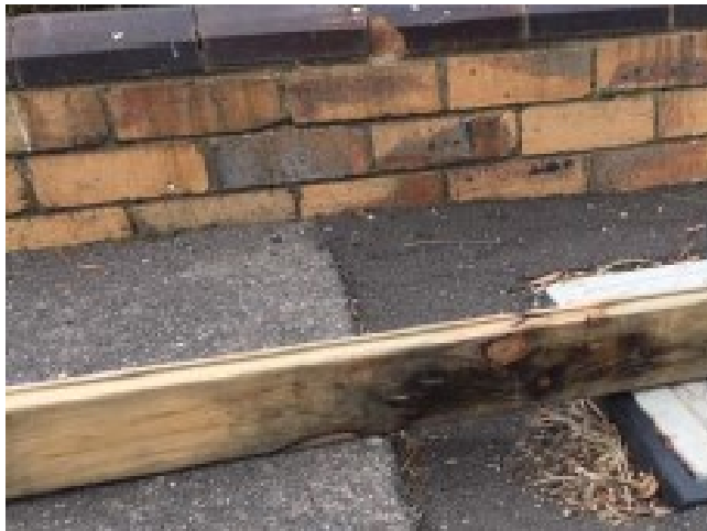
Figure 12: This reinstatement failed due to poor compaction of the subgrade layers and the top layer of asphalt. Resulting in a large lip against pit, causing a severe tripping hazard.
