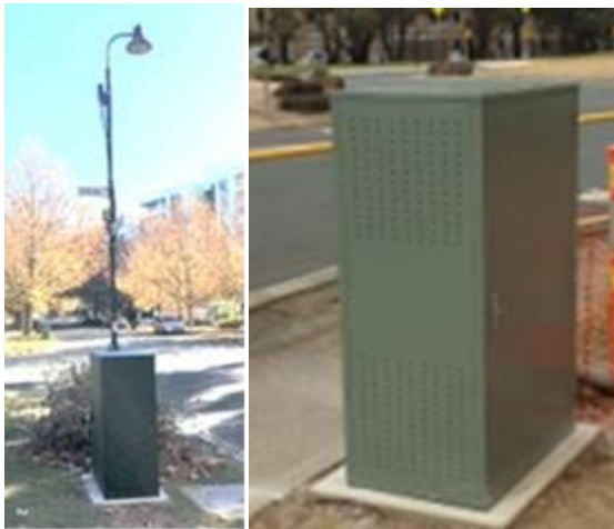
Figure B: In order to install a 5G antenna on one of the light poles (to which the council does not object) Optus have said they would also need to install a cabinet like the one below next to the pole. It is expected that the other carriers will soon arrive to put more cabinets next to the mall's other poles.
