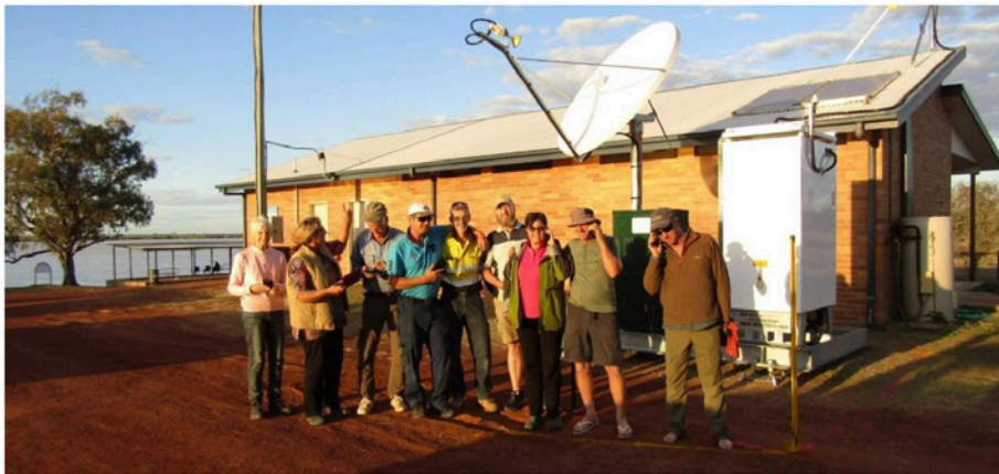
The Telstra 4G Mobile Satellite Small Cell tower being used by tourists at Lake Dunn.
