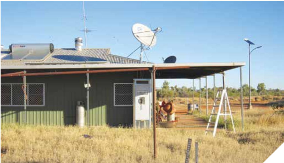
Building-mounted Wi-Fi phone installed at Labrapuntja. Image courtesy of Australian Private Networks Pty Ltd
