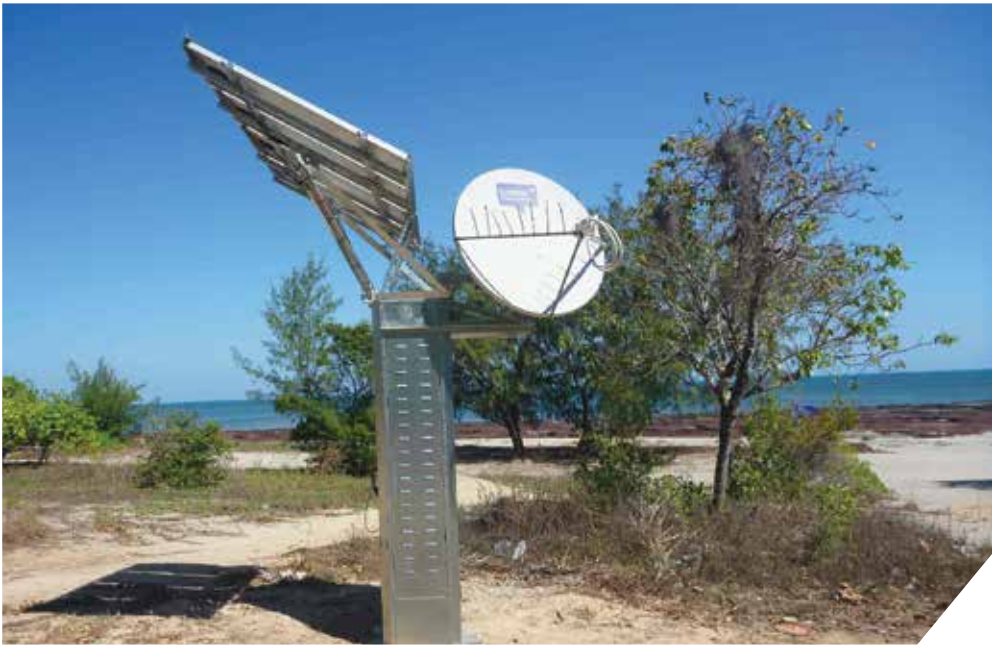
Freestanding Wi-Fi phone installed at Marramarrani. Image courtesy of Australian Private Networks Pty Ltd
