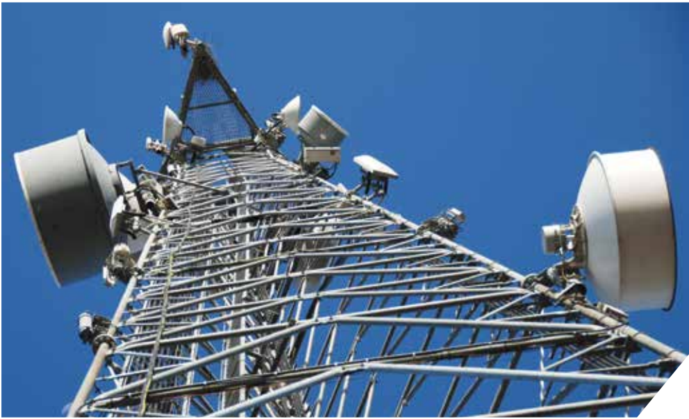
Communications tower with microwave dishes
