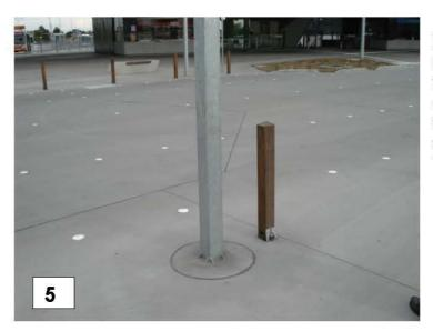
Photo 5 demonstrates the lack of clear demarcation between footpath and roadway as well as the lack of contrast between the pole and its background which clearly needs warning TGSIs to protect pedestrians. **Photo 6** Shows the "pedestrian crossing" on the eastern pedestrian approach to the station entrance presenting TGSIs that have been applied almost in compliance AS1428.4.1 creating a far safer entry/departure path for all pedestrians including those who are blind or vision impaired.
