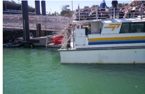
Nelly Bay gangways (pontoon ramps) serving upper and lower ferry decks
