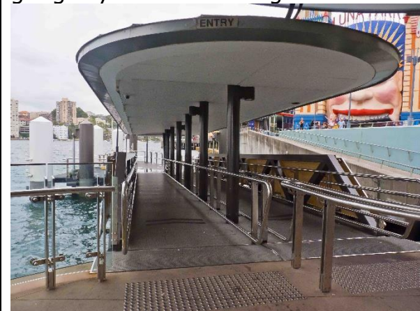
Milsons Point ferry wharf's new gangway has no landings
