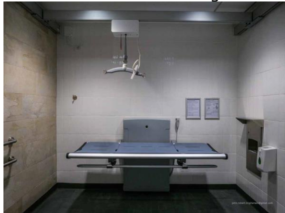
Adult adjustable height change table folded out and ceiling hoist
