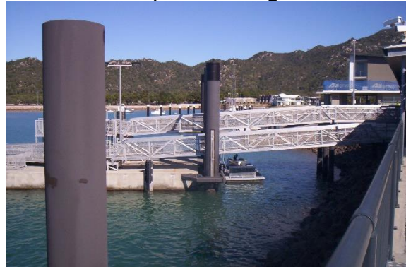
Nelly Bay gangways (pontoon ramps) that accommodate different ferry deck heights
