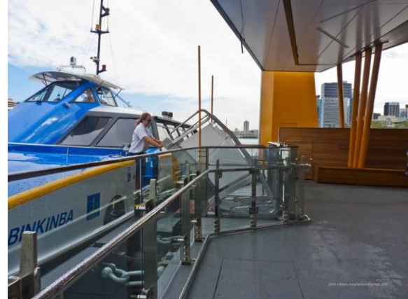
Nelly Bay gangways (pontoon ramps) serving upper and lower ferry decks
