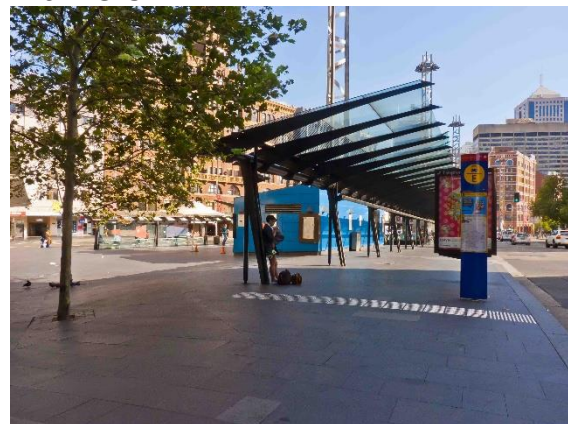
Railway Square Interchange boarding point blade lacks tactile markers
