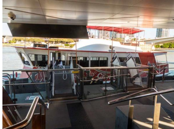
Nelly Bay gangways (pontoon ramps) that accommodate different ferry deck heights
