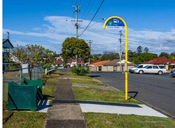
Steep slope and crossfall at the boarding point
