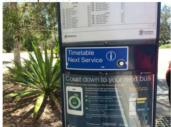
Next Service Console in bus stop blade showing height above boarding point
