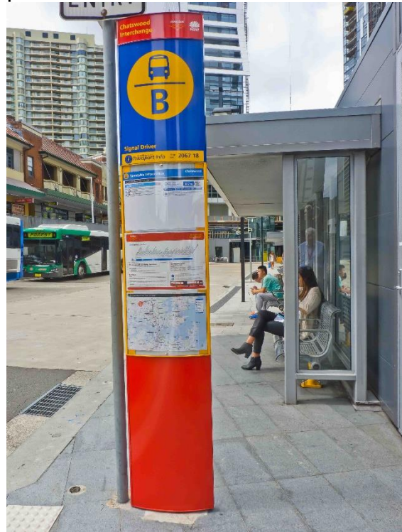
Railway Square Interchange boarding point blade lacks tactile markers
