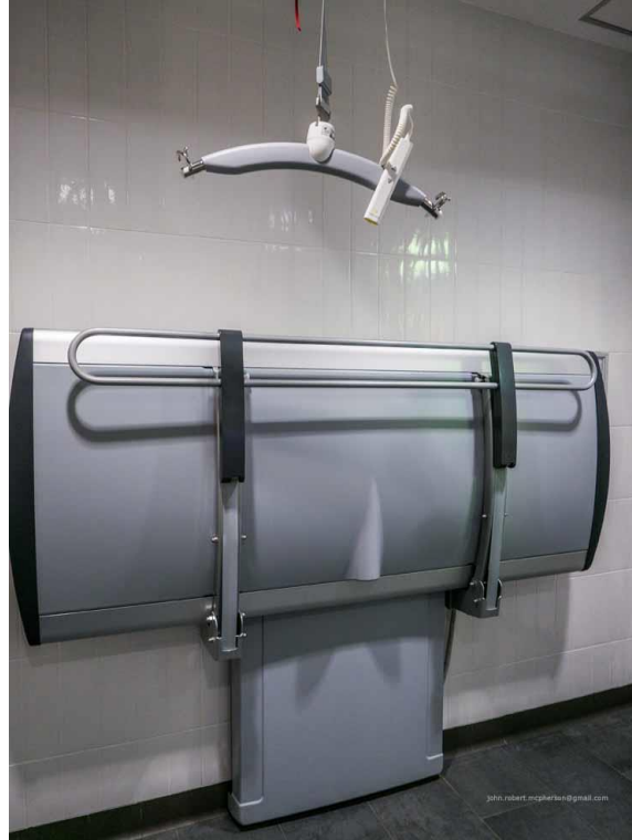
Adult adjustable height change table folded away and ceiling hoist
