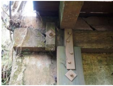
Deteriorated northern header beam
