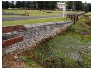
Settled downstream arch and headwall
