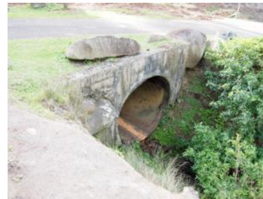
Outlet to upstream culvert
