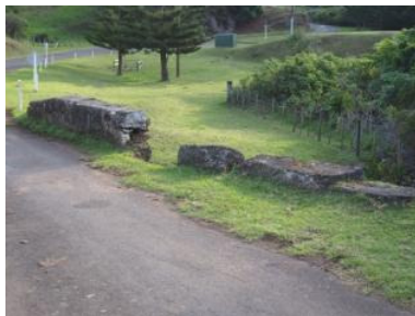
Damaged downstream headwall
