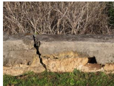
Damaged upstream headwall
