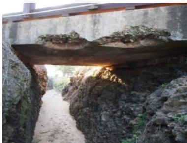
Corroded seaward slab edge.
