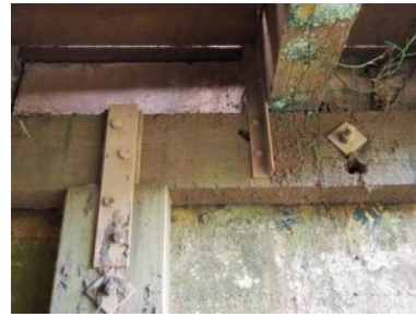
Deteriorated northern header beam
