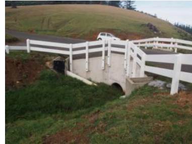
Road gullies discharging to drainage channel
