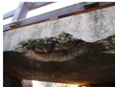
Steel Reinforcement now ineffective
