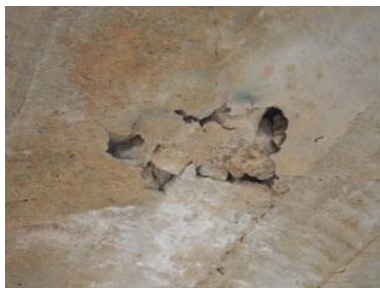
Poor quality concrete.
