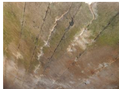
Cracks with calcification
