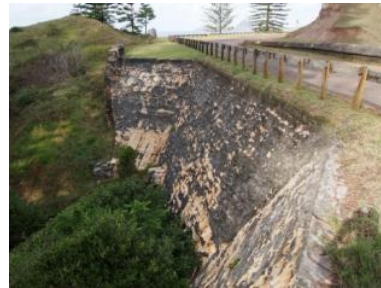
Splayed downstream wall
