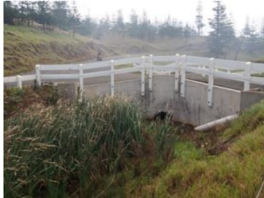
Culvert from downstream side
