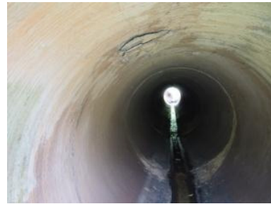
Damaged RC pipe culvert
