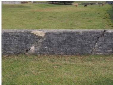
Cracked upstream headwall
