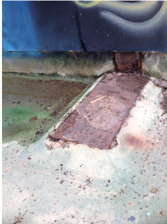
Photograph 13: Typical corrosion at base of columns in Eastern wall
