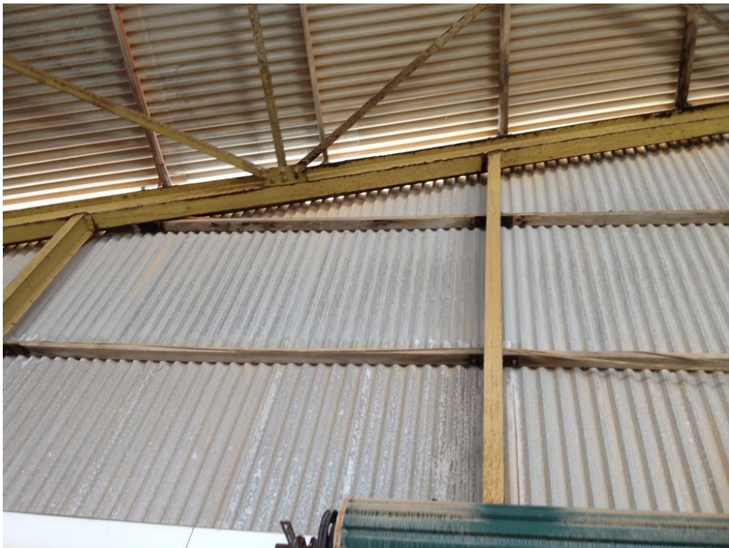
Photograph 10: Typical deterioration of paint finish and corrosion of exposed structural steel framing
