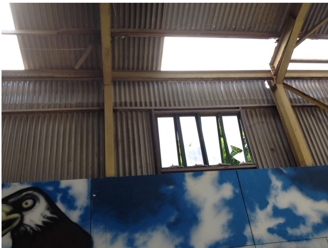
Photograph 7: Typical broken window panes at high level in Eastern wall
