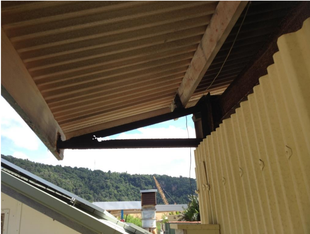
Photograph 5: Typical corrosion of structural steel eaves support framing
