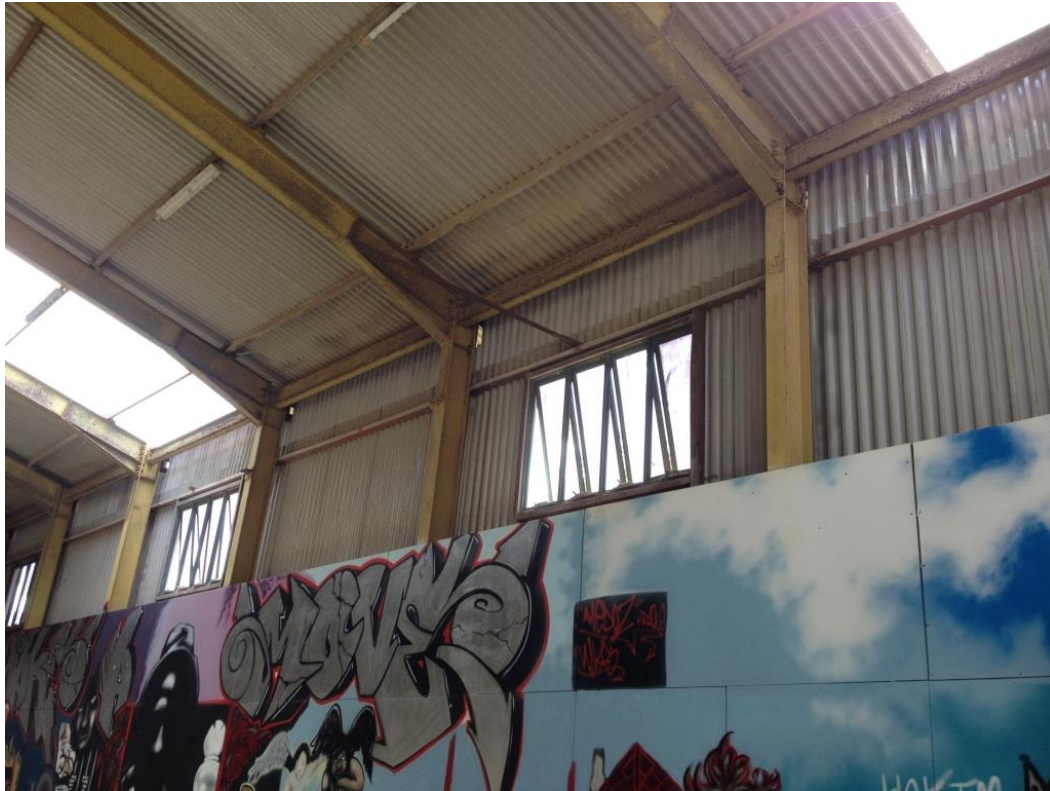
Photograph 9: Typical deterioration of paint finish and corrosion of exposed structural steel framing
