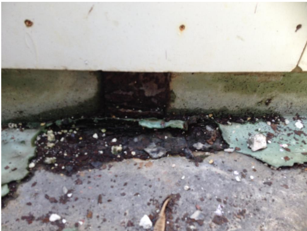
Photograph 14: Typical corrosion at base of columns in Northern and Southern walls
