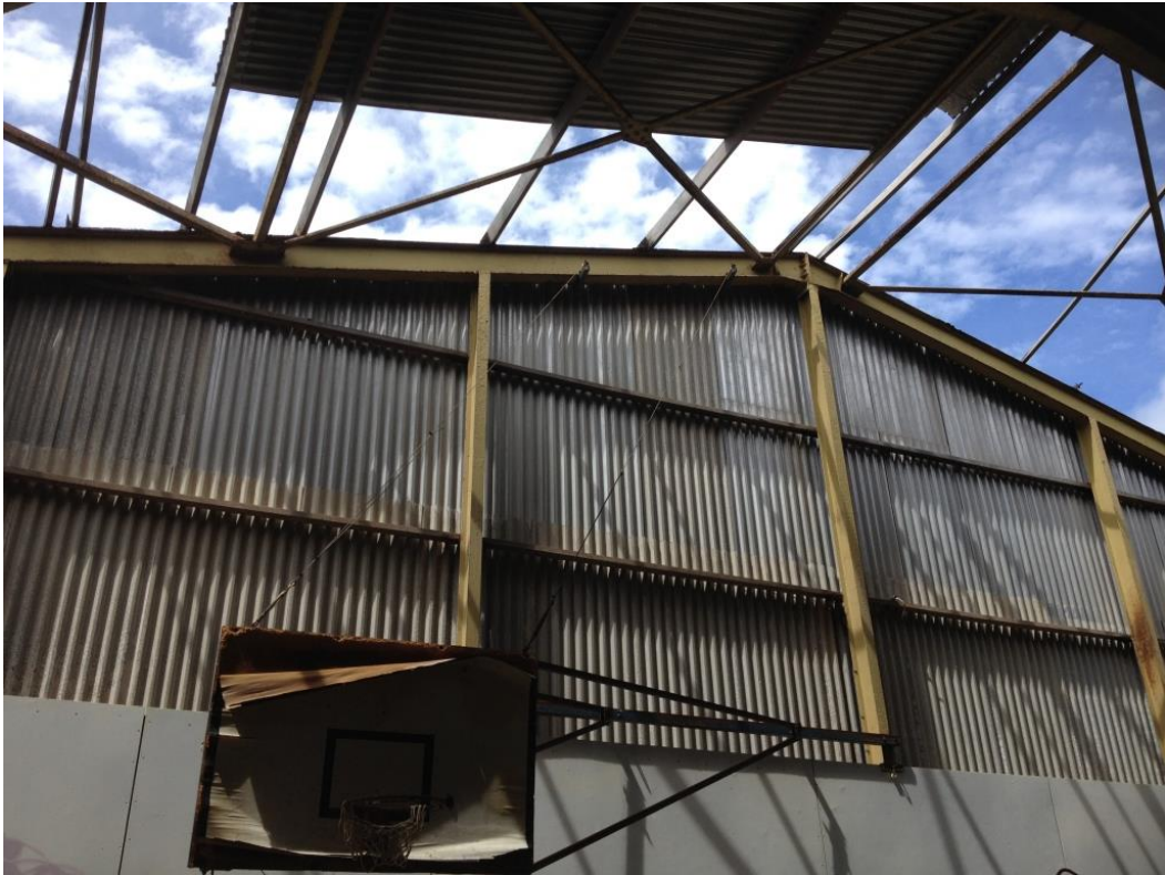
Photograph 1: Missing roof sheeting at Northern end bay of building
