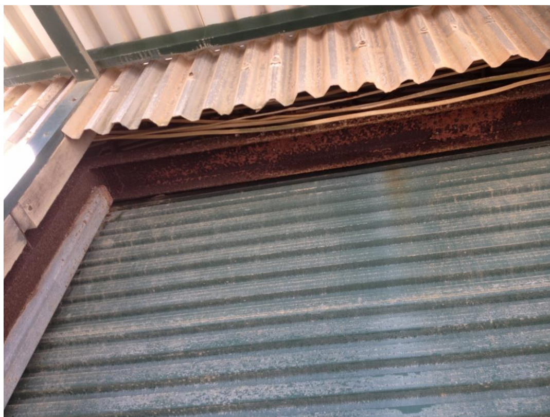
Photograph 8: Typical corrosion of exposed structural steel framing at roller shutter doors
