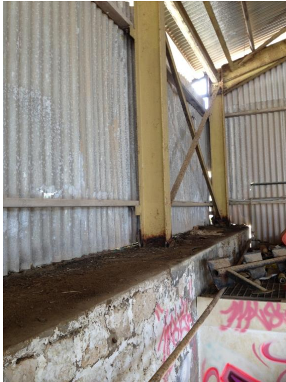
Photograph 11: Typical corrosion of at base of columns at Western wall
