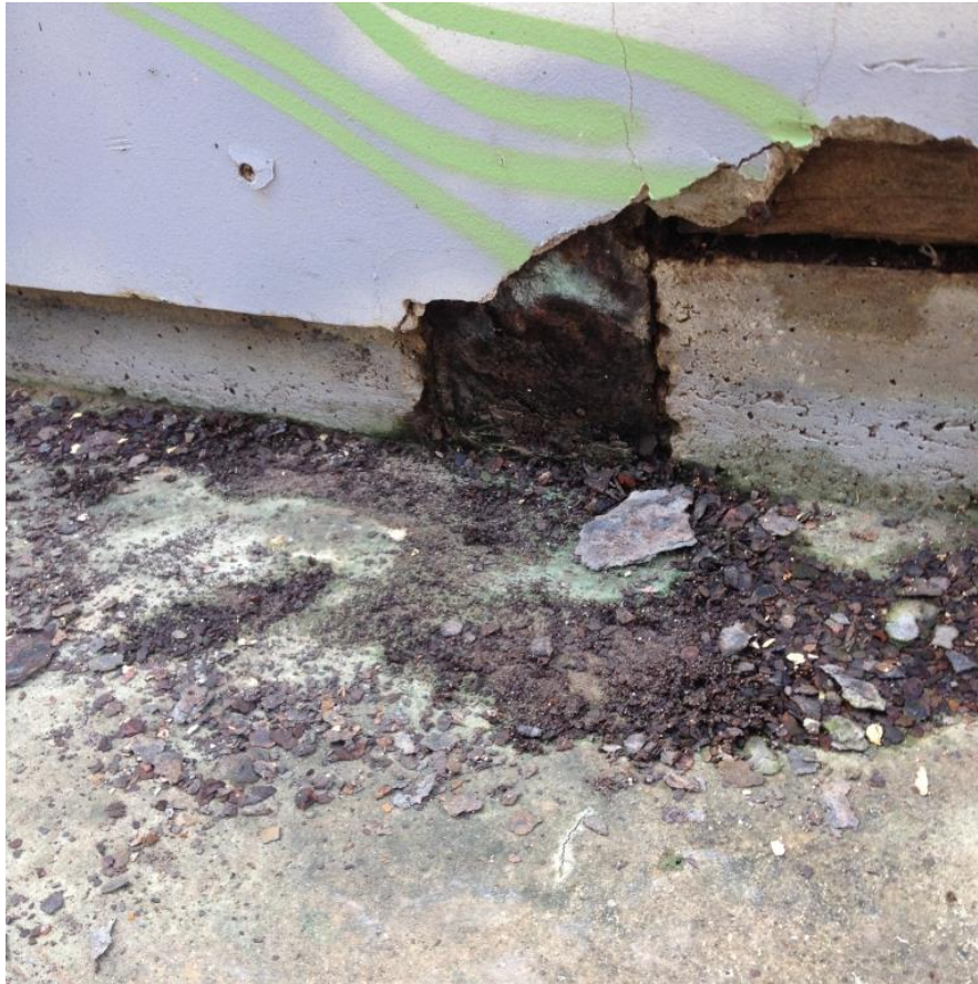
Photograph 15: Typical corrosion at base of columns in Northern and Southern walls
