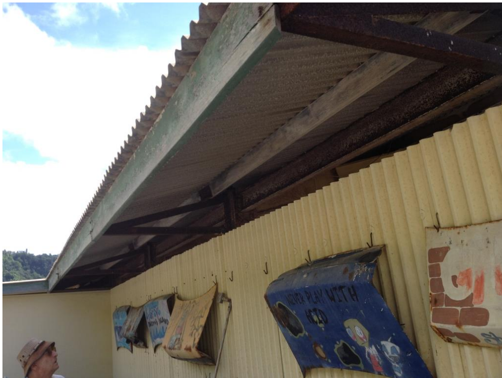
Photograph 6: Typical weathering and corrosion at eaves support framing
