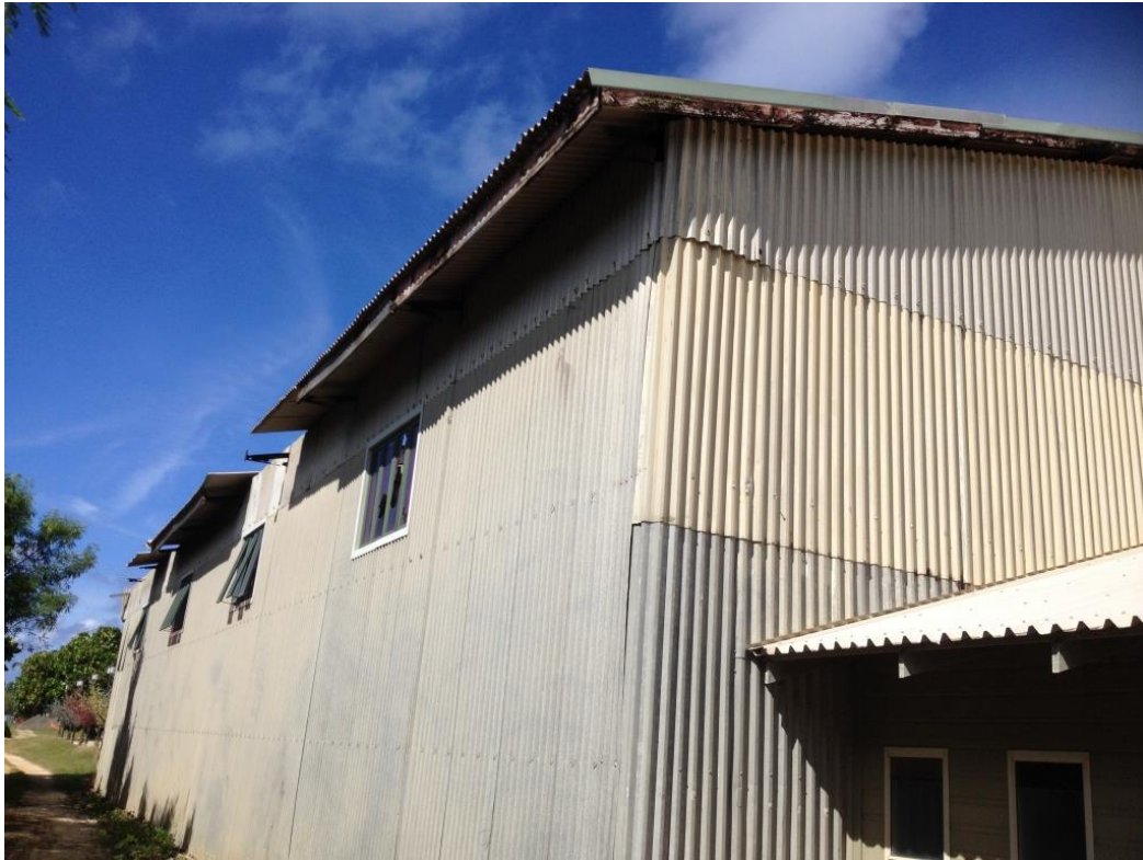
Photograph 3: Sections of missing eaves cladding and structure along Eastern wall
