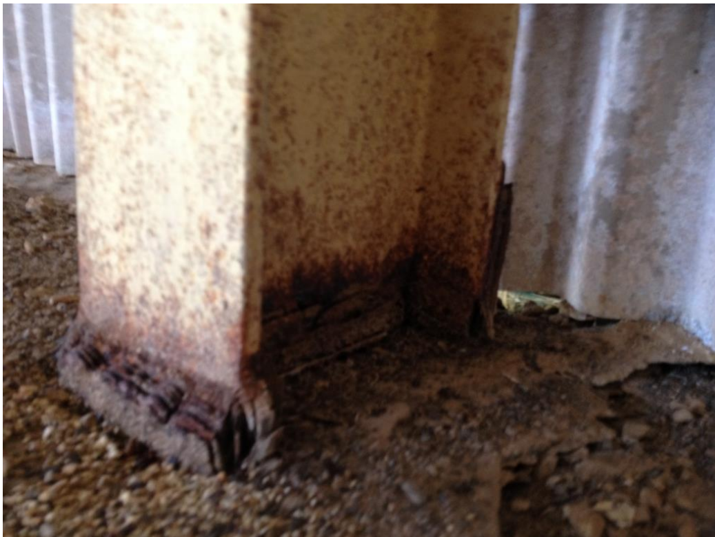
Photograph 12: Typical corrosion of at base of columns at Western wall
