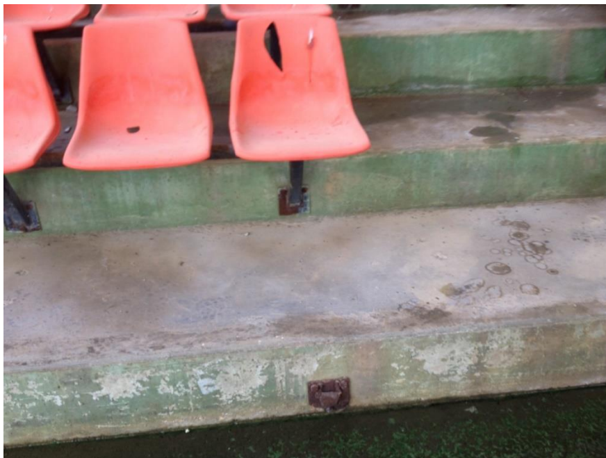
Photograph 16: Damage to plastic seats and corrosion of support framing
