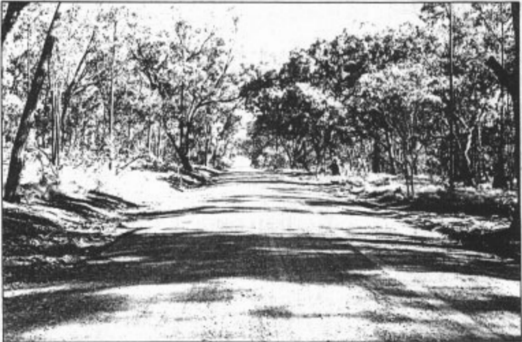
Site 24 - Undivided, 2-Lane, Gravel wide, Walled road.
