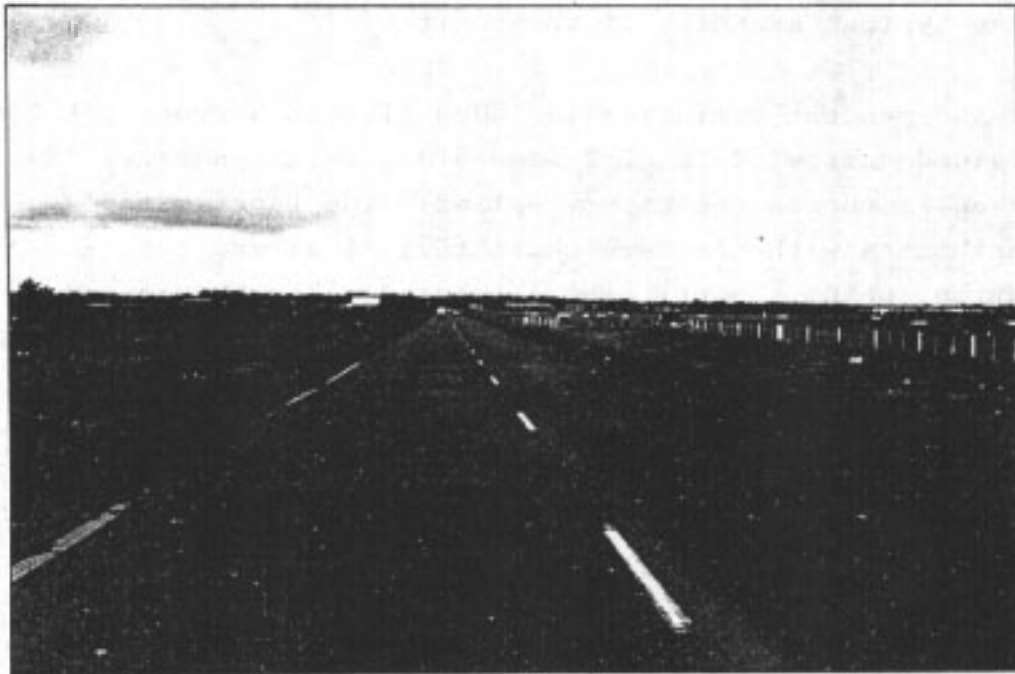
Site 45 - Undivided, 2-Lane, Narrow, Spacious road.
