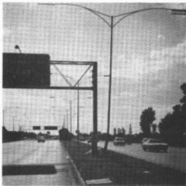
Figure 17 An unnecessarily rigid luminaire support on a freeway median.
