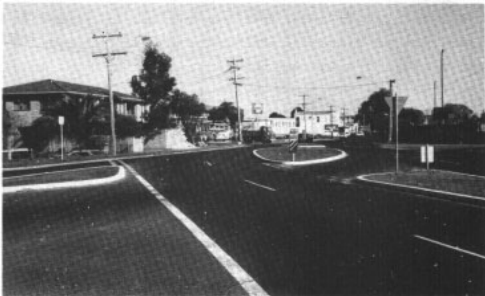
Figure 12 A combination of curvature, incorrect camber, low skid resistance and corrugations in the road surface caused seven pole accidents in eight months at this site. The predictor model developed in this study allows identification of such high risk sites and the nature of the required remedial action.
