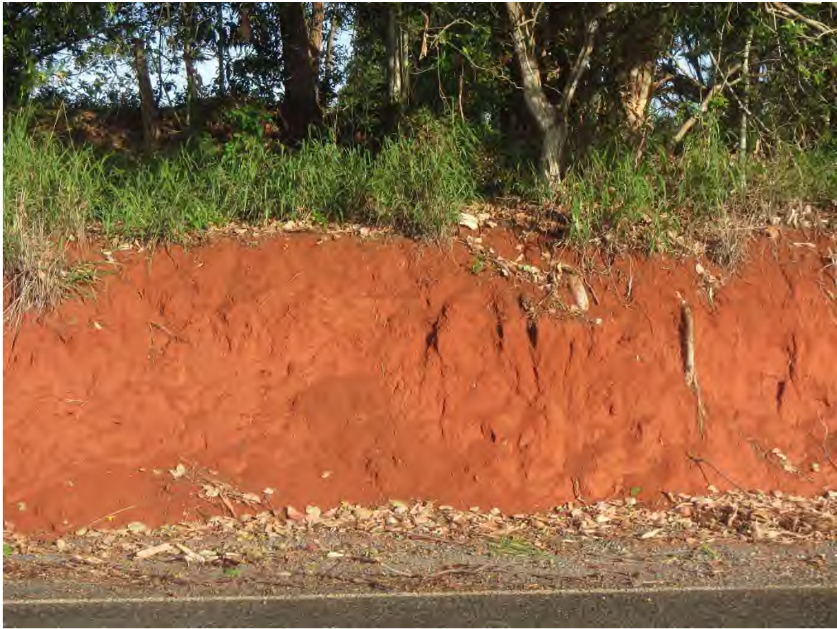
Photograph 7: Cut 4 (LHS) - Residual soil batter
