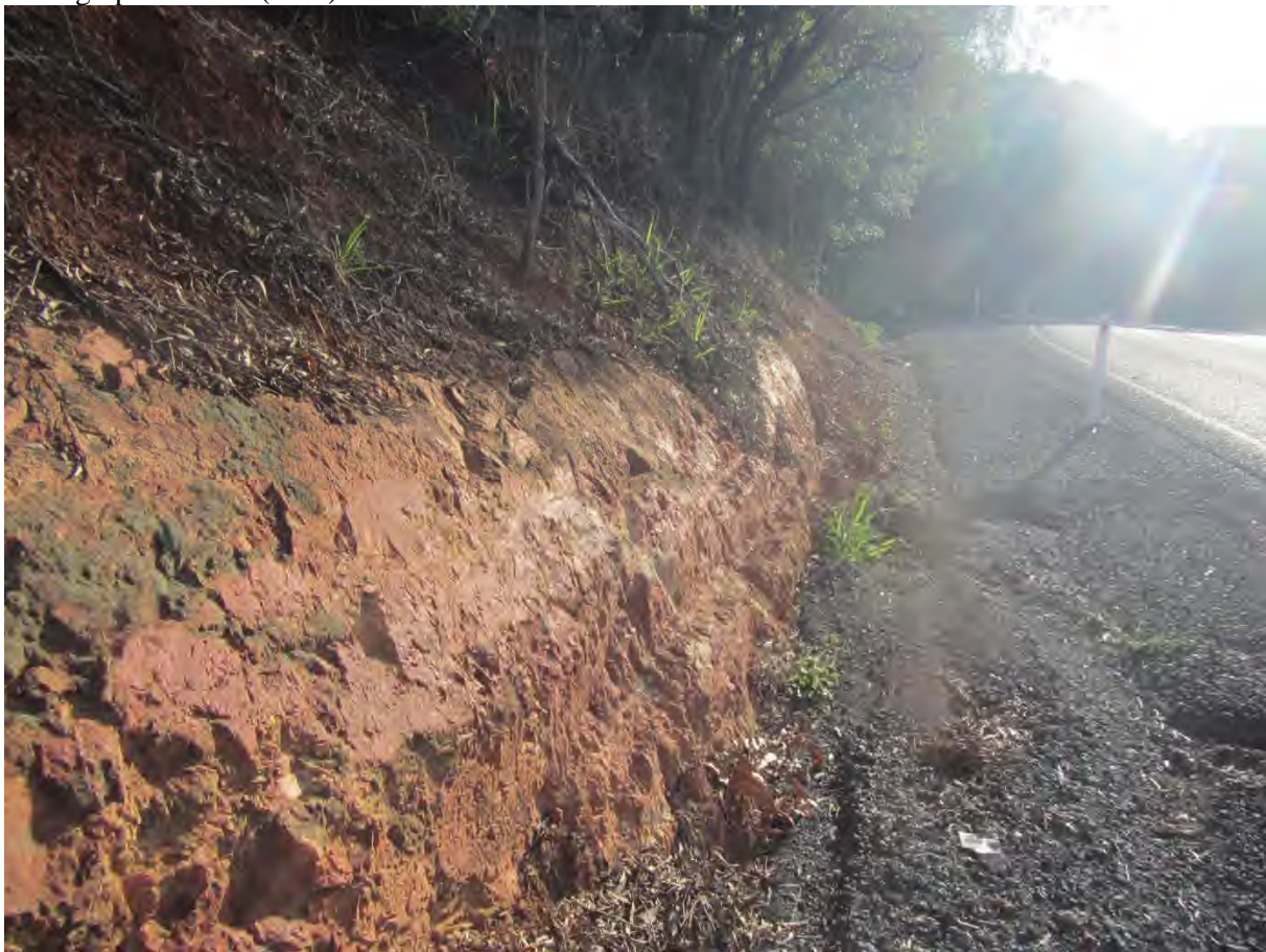
Photograph 6: Cut 3 (LHS) - MW Siltstone
