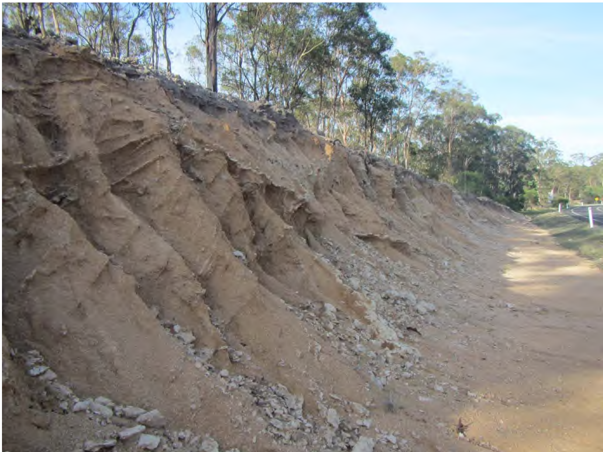
Photograph 2: Cut 1 (RHS) - Rilling erosion in XW granite
