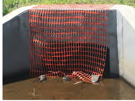
Figure 15. Ineffective measures to exclude birds from culverts should be avoided. Where possible, exclusion devices should be permanent, and ideally incorporated into culvert design.
