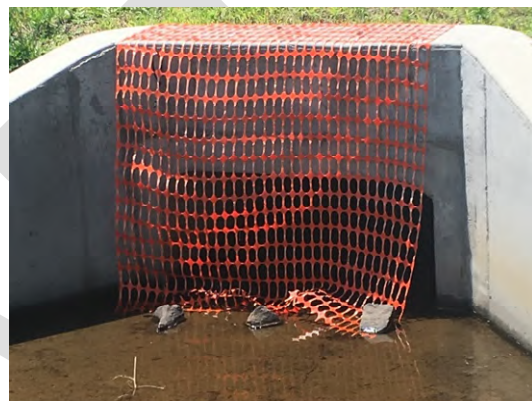
Figure 19. Ineffective measures to exclude birds from culverts should be avoided. Where possible, exclusion devices should be permanent, and ideally incorporated into culvert design.
