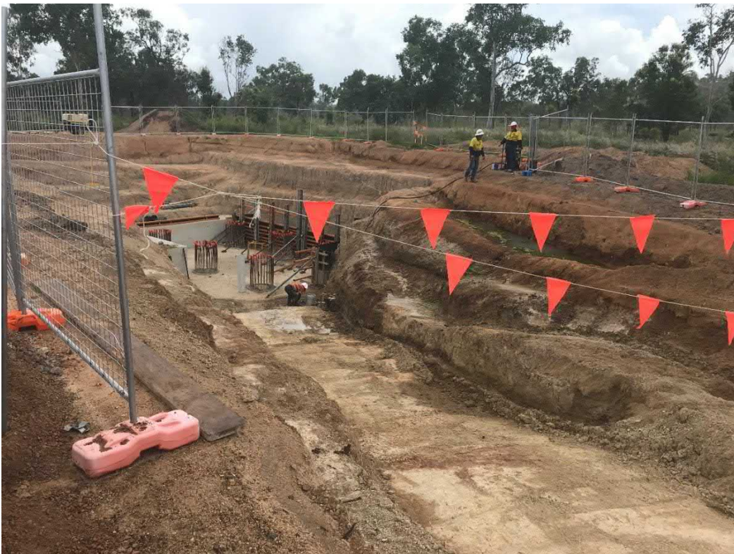
Plate 9 Stage 1 Thrust Excavation for QR Railway Underbore (Package 4)
