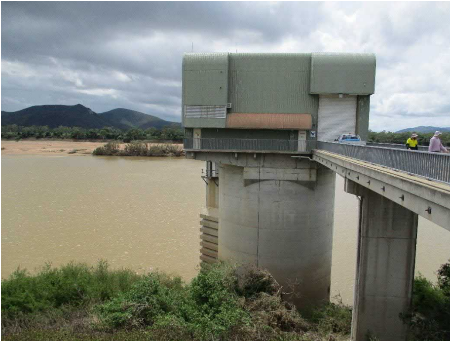
Plate 17 Existing Sunwater Tom Fenwick Intake and Pumping Station
