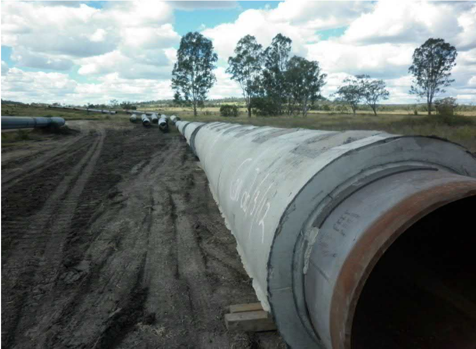
Plate 13 Example of Reactive Soils at Pipeline Inverts
