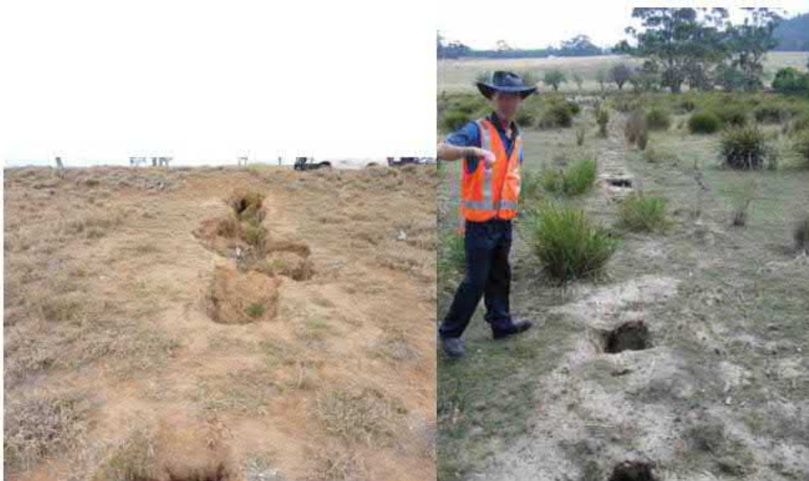
Plate 15 Typical Tunnel Erosion of Over Pipeline Backfilled Alignments
