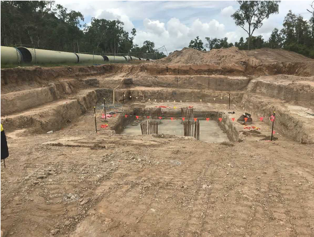
Plate 7 Stage 1 Pipeline Thrust Block Excavation in Weathered Rock Sequences
