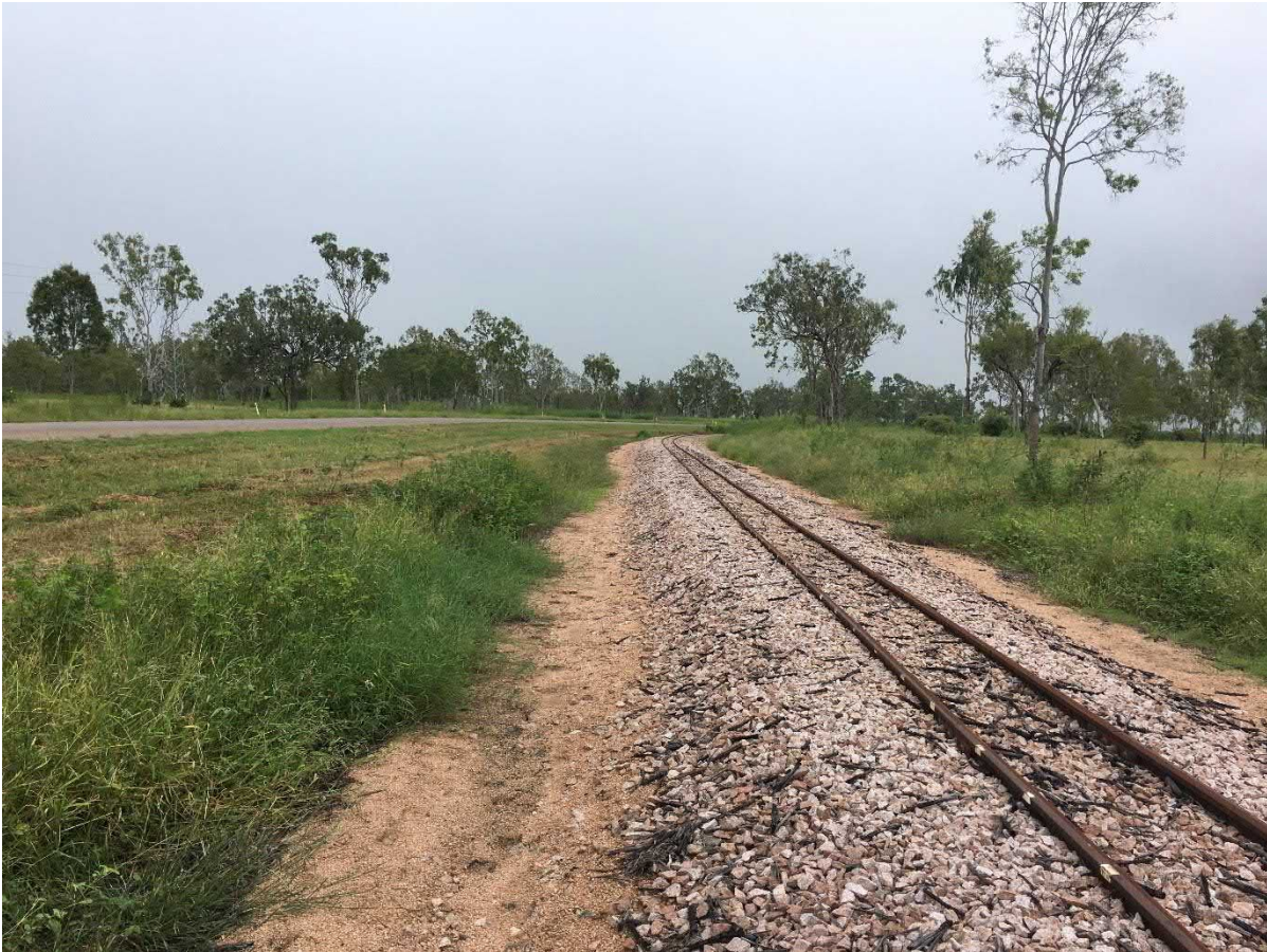
Plate 3 Typical Cane Railway Formation Within the Region
