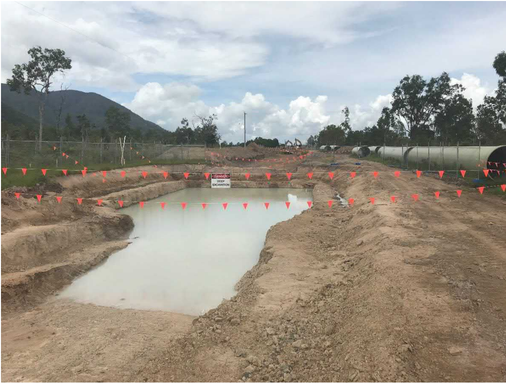
Plate 9 Stage 1 Thrust Excavation for QR Railway Underbore (Package 4)
