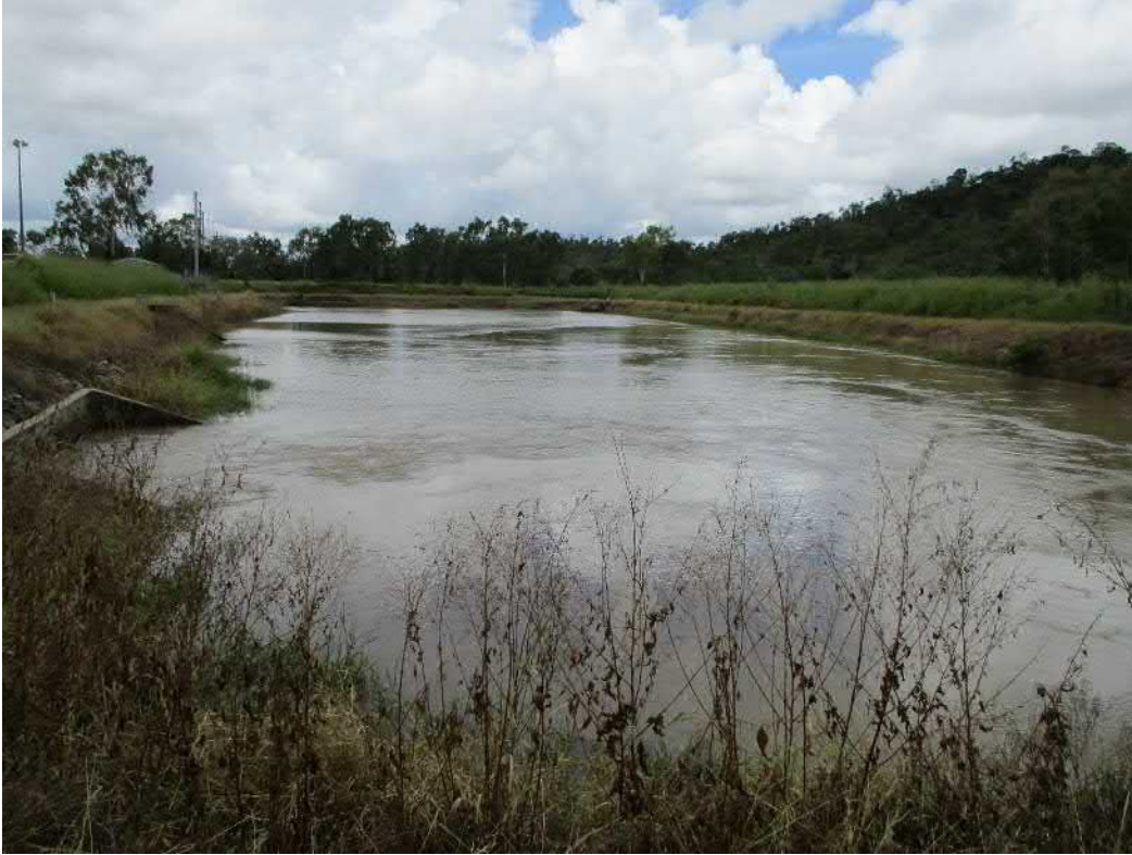
Plate 18 Existing Sunwater Tom Fenwick Surge/Balancing/Sedimentation Dam
