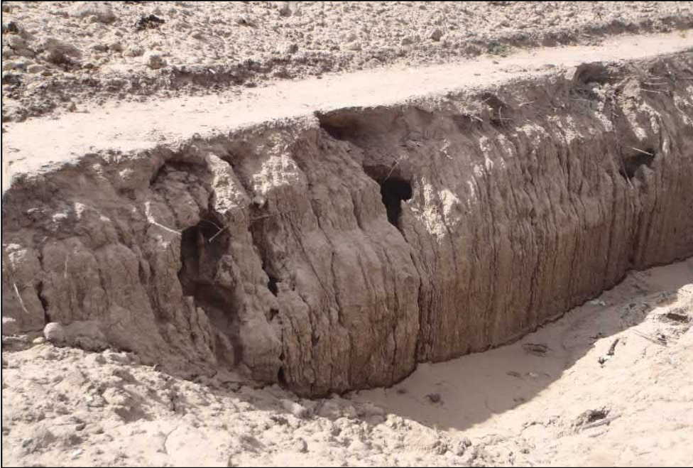
Plate 15 Typical Tunnel Erosion of Over Pipeline Backfilled Alignments
