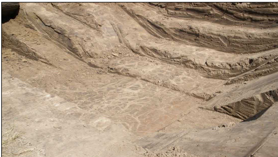
Plate 13 Example of Reactive Soils at Pipeline Inverts
