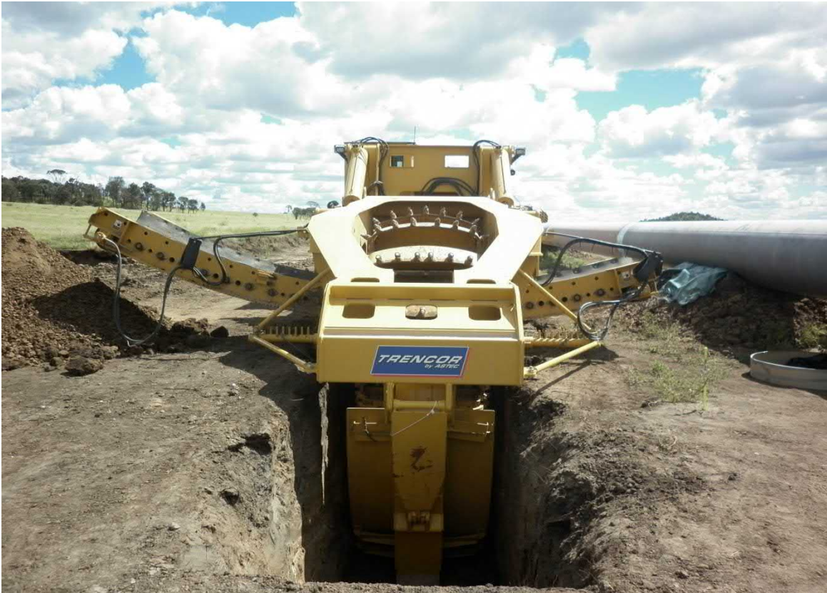
Plate 10 Typical Trenching Machinery Used in Large Diameter Pipeline Installation
