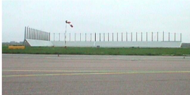
The so-called “**7-knots criterion**” was given further status via a follow-up study by Nieuwpoort et al (2006) based on flight simulations. The **BI-Wsh** rule developed through these studies was related to the maximum allowable lateral wind speed deficit occurring behind an obstacle:
