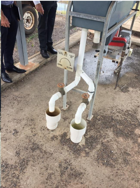
Photo 56. View of ARFFS station separator with storm water and sewer valve options.
