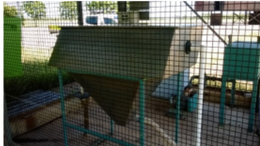
Figure 1 - HFTG coalescing plate separator
