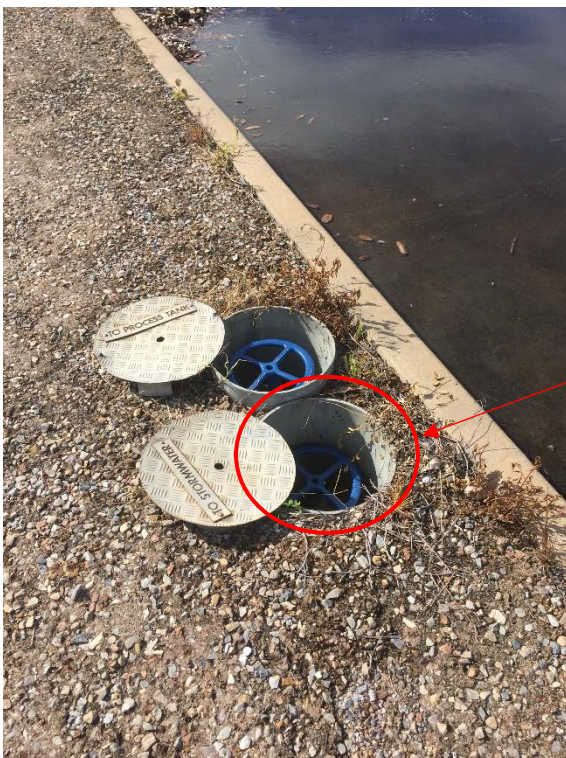
Photo 7. Close up view of release valves at LMU training ground. Note blue wheel is still attached to the storm water valve.
