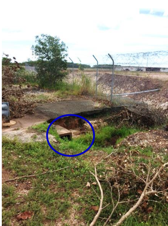
Photo 27. View of end of road storm water drain entering large storm water drain.
