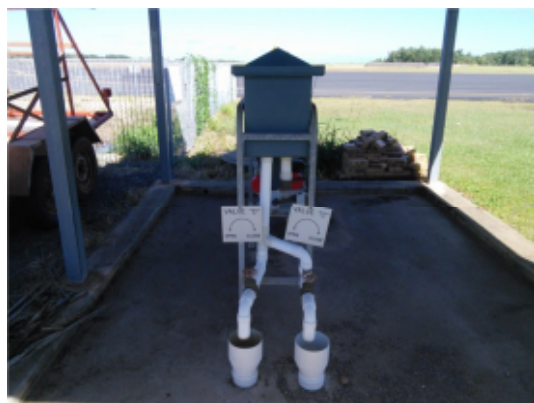
Figure 3 - ARFF Station coalescing plate separator
