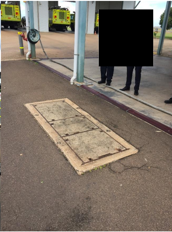
Photo 35. Close up view of triple interceptor.
