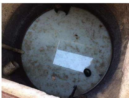
Figure 10 – Separator feed pit
