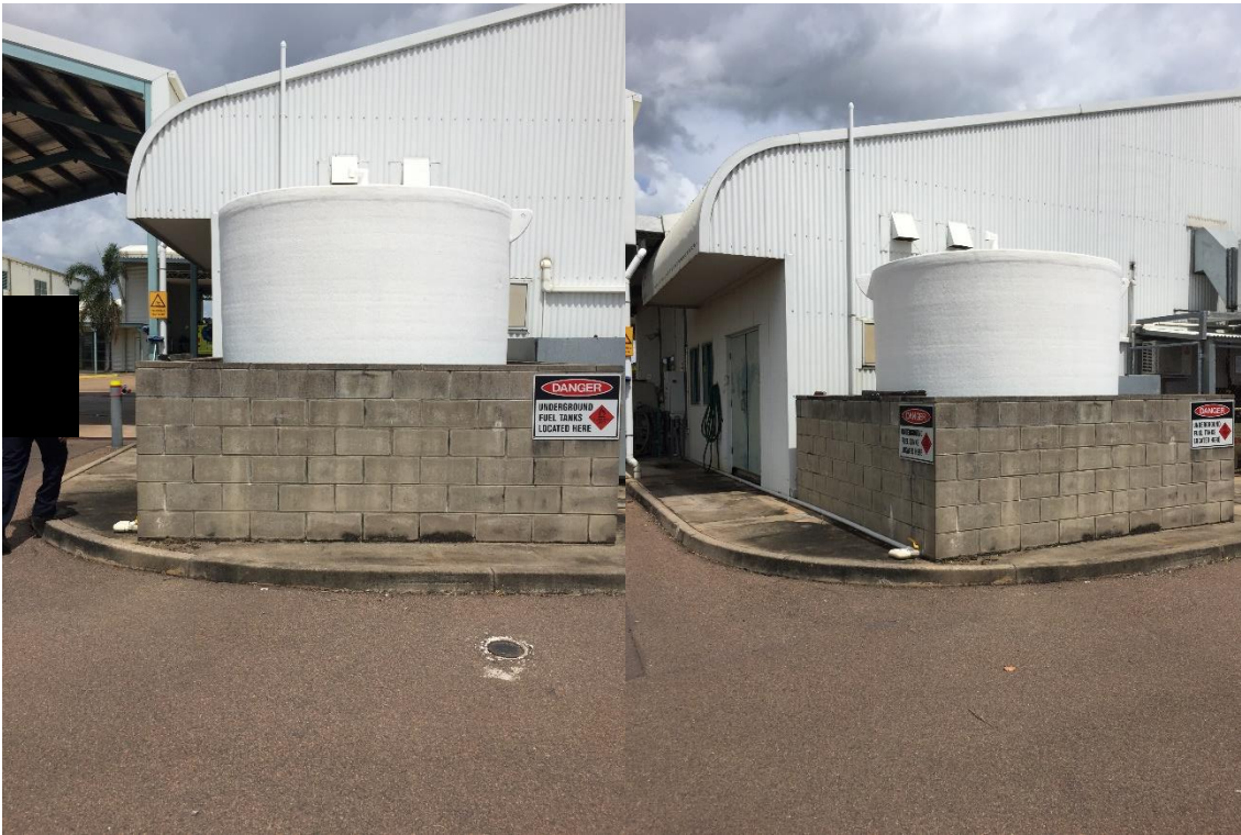
Photo 59. View south of ARFFS station bulk tank. Photo 60. Overall view of foam storage tank with retention wall.
