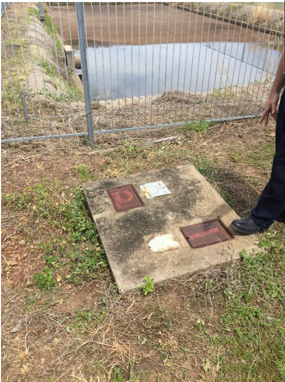
Photo 53. View of valves for ARFFS station retention pond. One valve is for storm water and the other is for diversion to the Underground Storage Tank (UST). Photo taken at northern end of the retention pond looking south.
