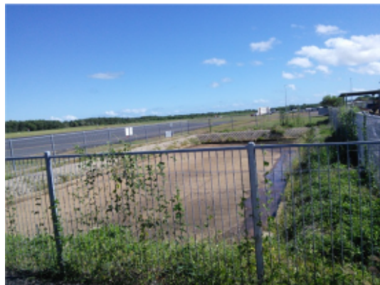
Figure 2 - ARFF station evaporation pond
