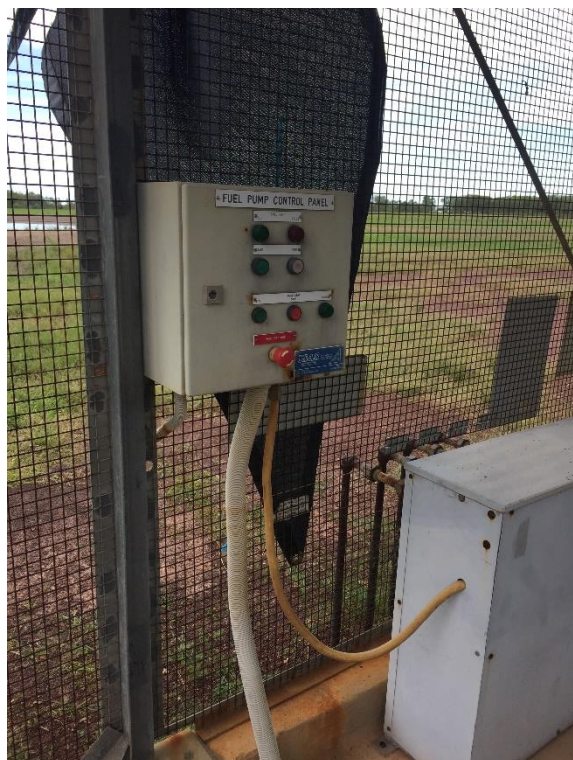
Photo 75. ARFFS LMU Defence training ground close up view of fuel pump panel and fuel lines exiting storage shed.
