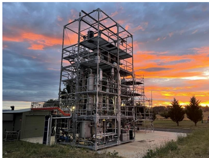
Above: SEATA Pilot Facility - Clean Energy and Carbon Sequestration R&D Centre, Glen Innes NSW (New England REZ).
