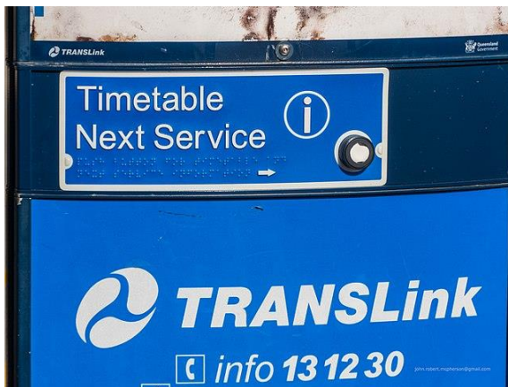
Close up of console with braille and tactile text embedded in boarding point blade, Chermside bus interchange, Brisbane.
