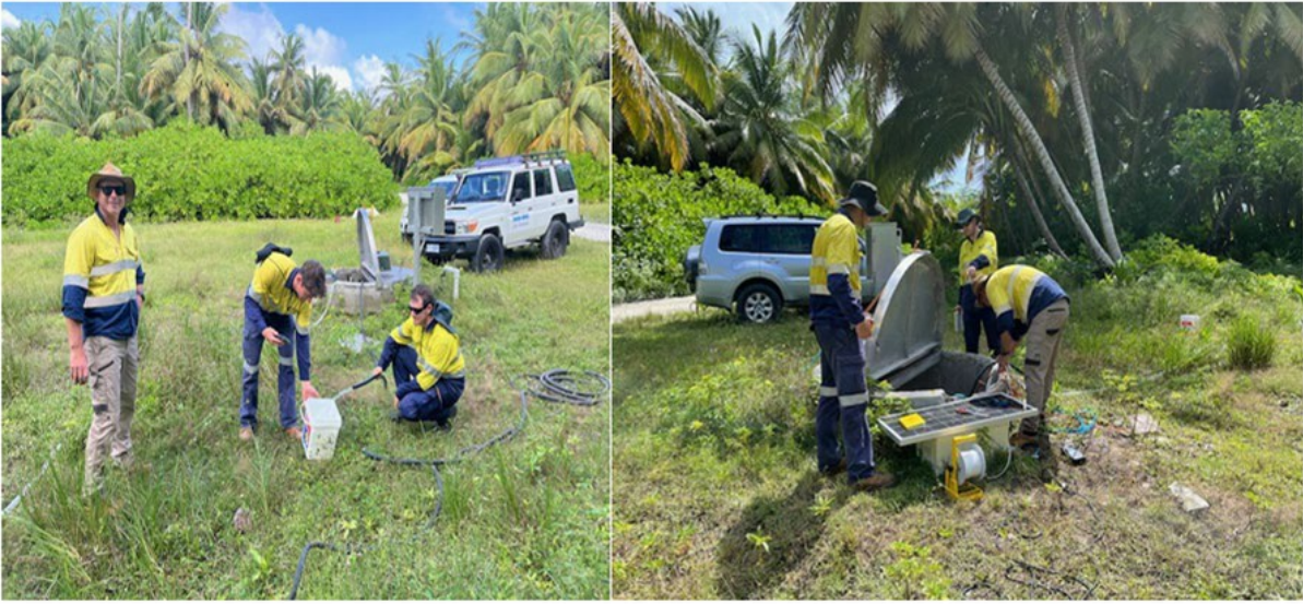
Image: DWER staff pump testing the HB3 water gallery
