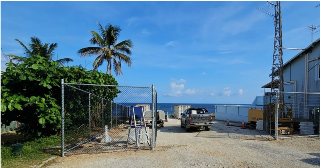
Image: CI AFP building after replacement of the fencing
