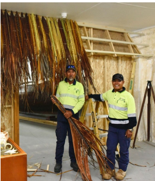
Image: Shire carpenters at work on gallery construction - Pulau Cocos Museum
