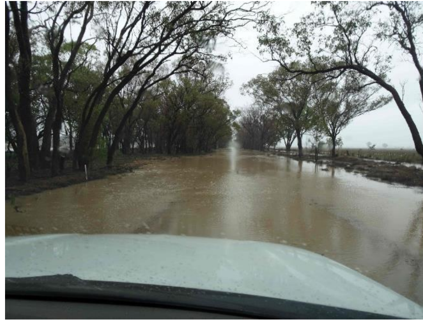
N2B green field alignment - Wallaby Rd 5 th March 2020 – 68 mm of rain over 48hrs (BoM: Dubbo AWS gauge No. 065070). Extensive alignment flooding to 50cm depth, velocity range 0.5 to 1.5 meters per second.
