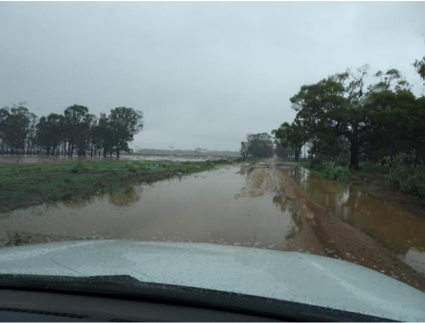
N2B green field alignment - Wallaby Rd 5 th March 2020 – 68 mm of rain over 48hrs (BoM: Dubbo AWS gauge No. 065070). Extensive alignment flooding to 50cm depth, velocity range 0.5 to 1.5 meters per second.
