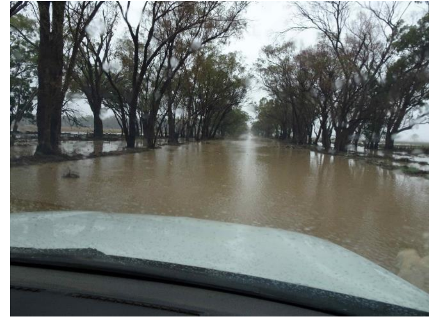
N2B green field alignment - Wallaby Rd 5 th March 2020 – 68 mm of rain over 48hrs (BoM: Dubbo AWS gauge No. 065070). Extensive alignment flooding to 50cm depth, velocity range 0.5 to 1.5 meters per second.
