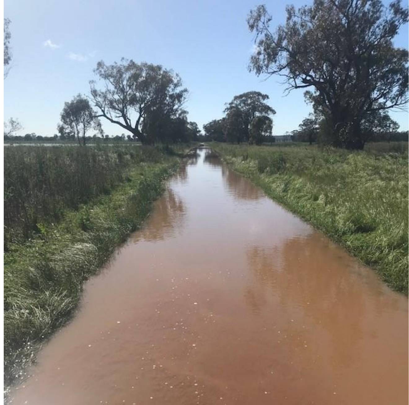
N2B Wallaby Rd & Dappo Rd 9 th Oct 2022 – 106 mm over 5 days (BoM: Dubbo AWS gauge No. 065070). Images 10 hrs after peak flow, flood depth and velocity too dangerous to proceed.
