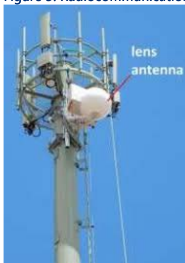
Figure 3: Radiocommunications lens antenna
