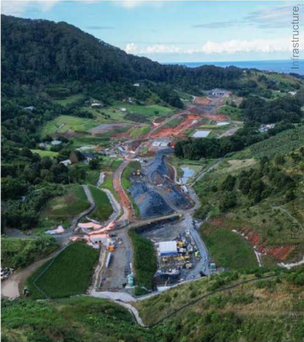
Coffs Harbour Bypass: Mackay Road, looking west4 July 2025
