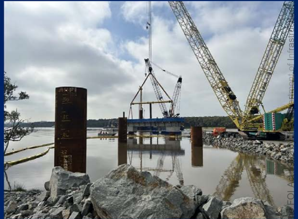
M1 to Raymond Terrace: Bridge 5 (Viaduct) pile cap shell installation from Hunter River rock platform – March 2025
