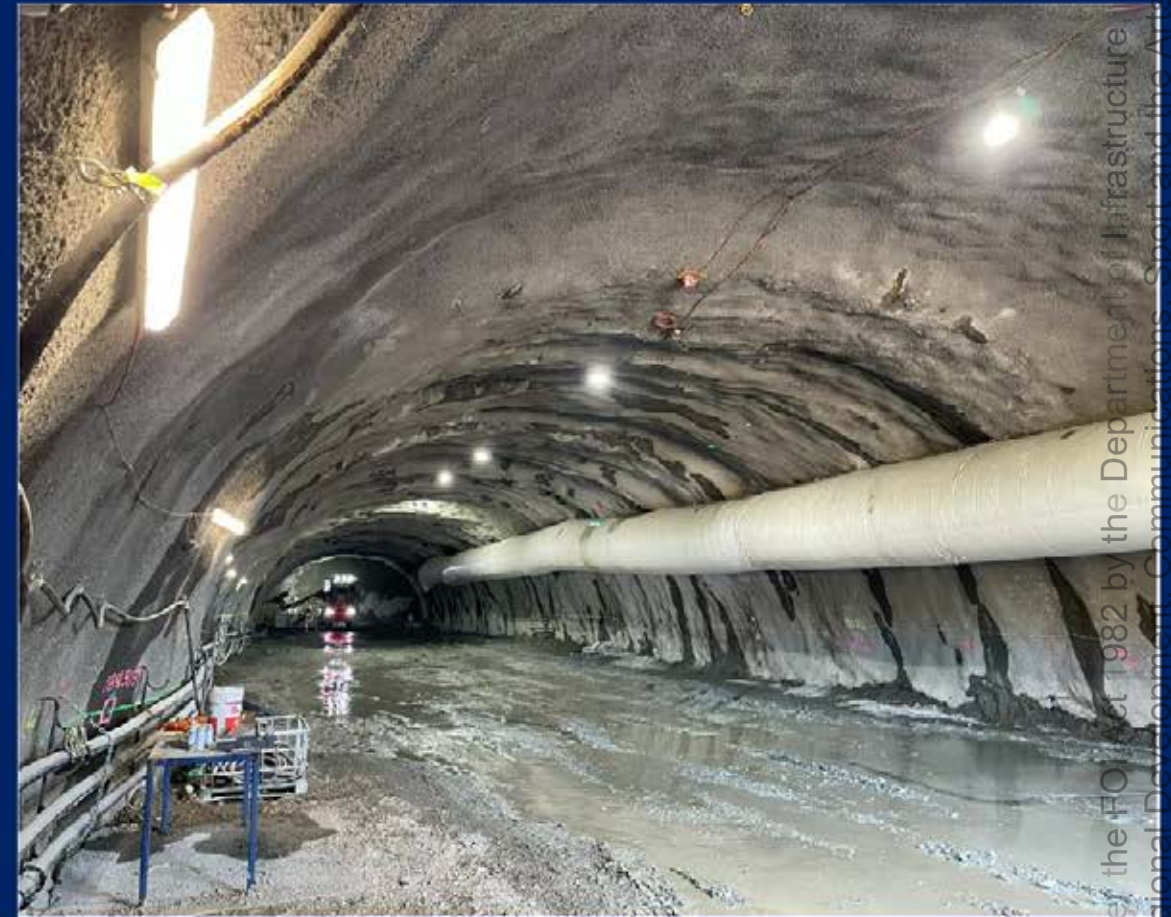
Coffs Harbour Bypass: Gatelys tunnel, Jun-24
