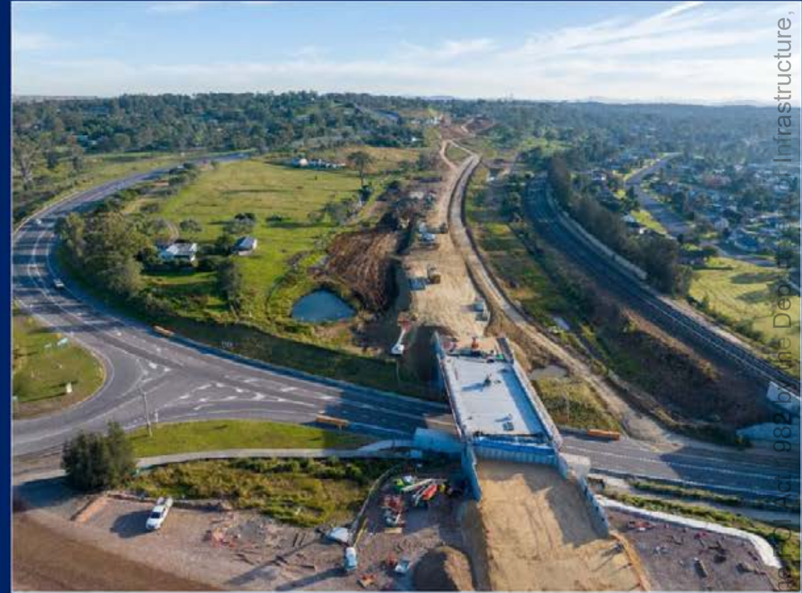
Singleton Bypass – Bridge over New England Highway at Gowrie Northbound – June 2025
