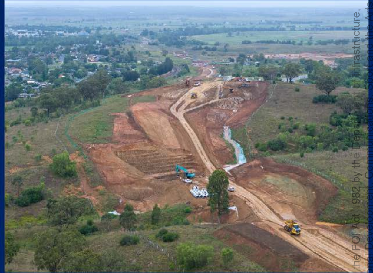
Singleton Bypass: Earthworks at McDougalls Hill, looking southbound – Jan 2025
