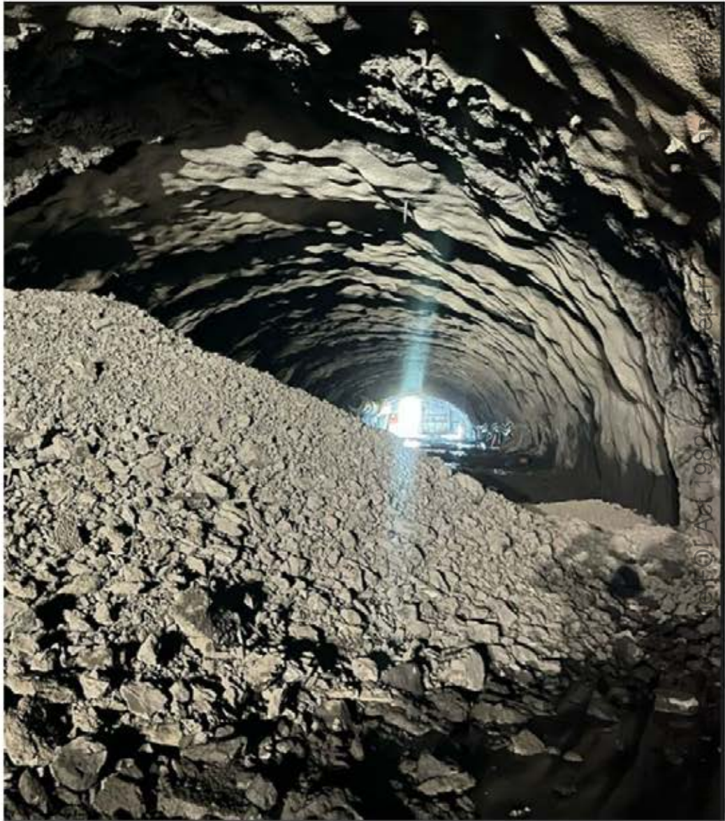
Coffs Harbour Bypass: Shephards Lane tunnel, 4 southbound breakthrough – 31 March 2025
