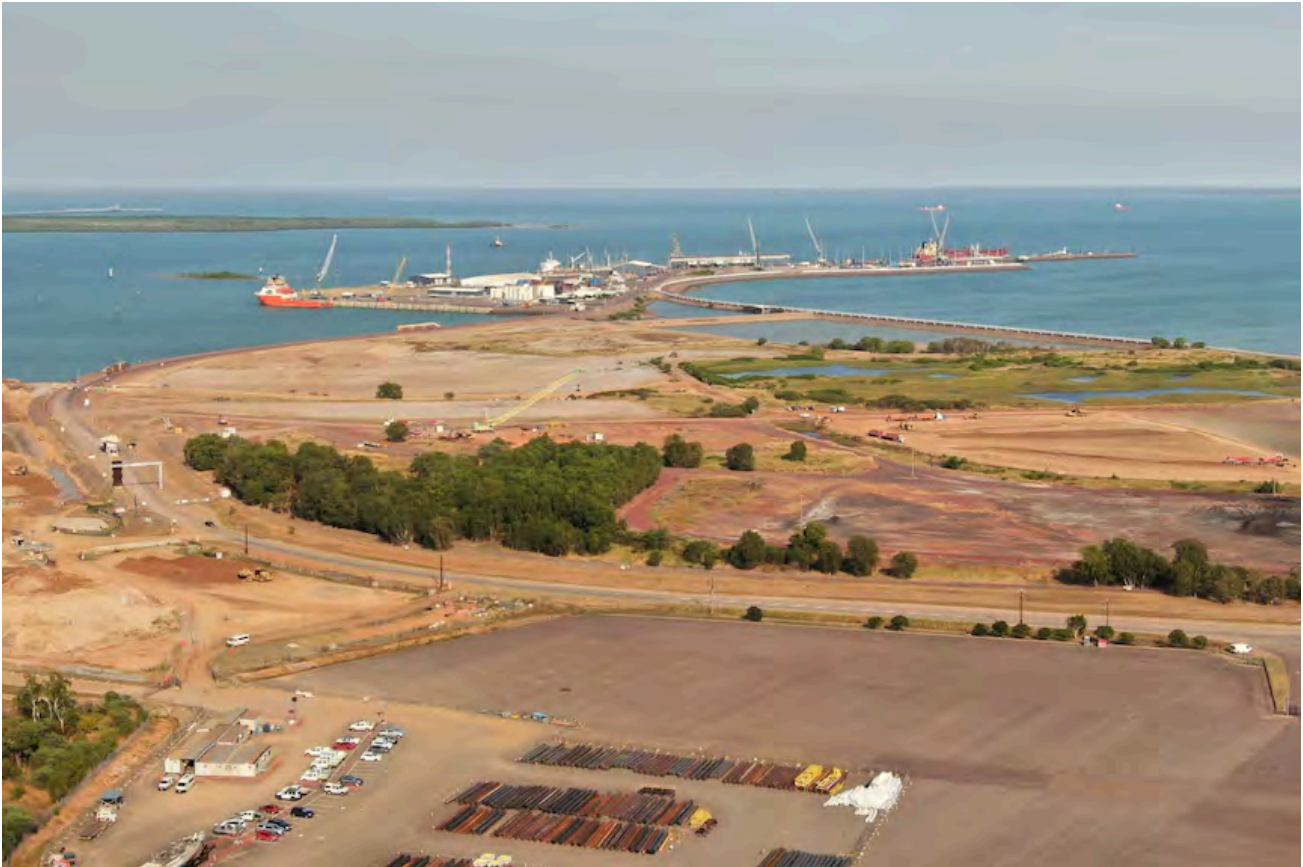
A potential site for 16 storage tanks has been identified at East Arm. (ABC News: Dane Hirst)
