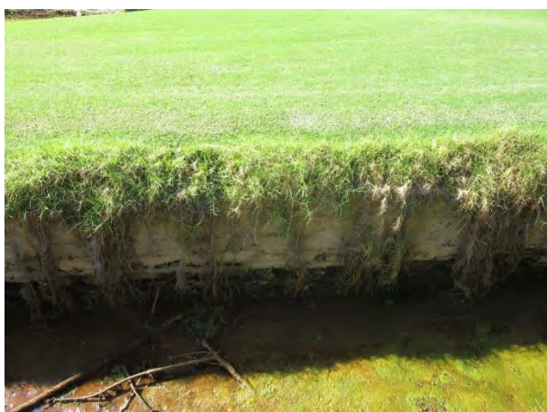
Figure 15: Concrete lining at West end of the 1941 channel
