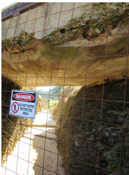
Figure 23: Bridge deck from 1941 channel
