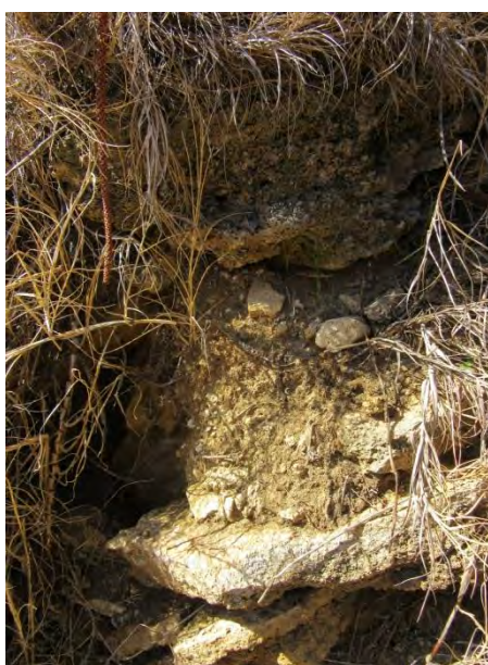
Figure 21: East end of the 1941 channel walls showing bedding
