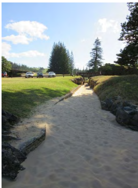
Figure 6: 1941 channel from East
