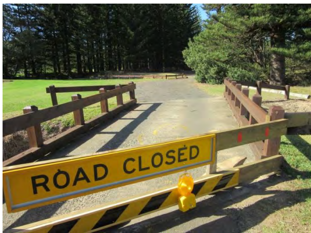
Figure 20: Bridge deck looking East
