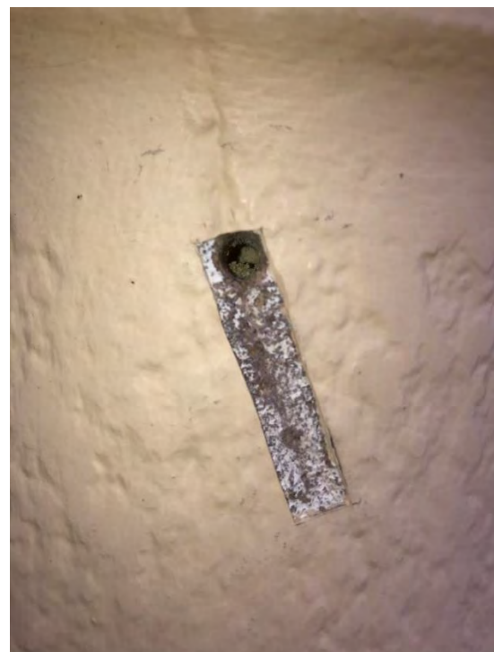
Figure 15 Upper Groove with Drill Hole
