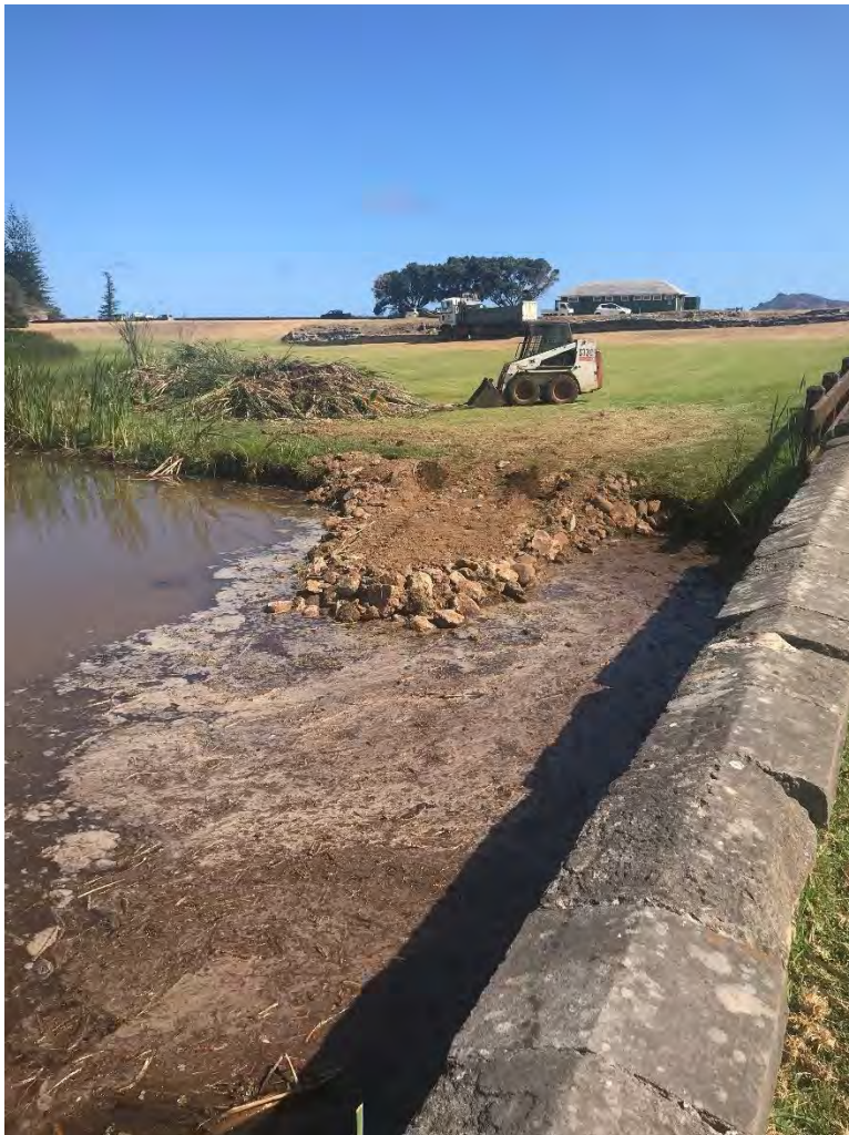
Figure 5 Construction of Coffier Dam
