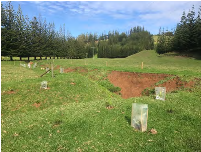
14. Ongoing erosion of banks by cattle accessing the creek for water, damage exacerbated by storm water flow scour, increasing the depth of the creek bed and further eroding its banks
