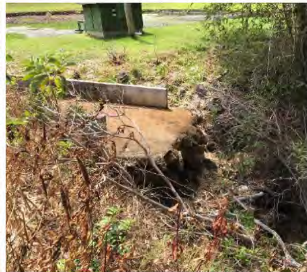
Figure 17 Downstream end of spillway
