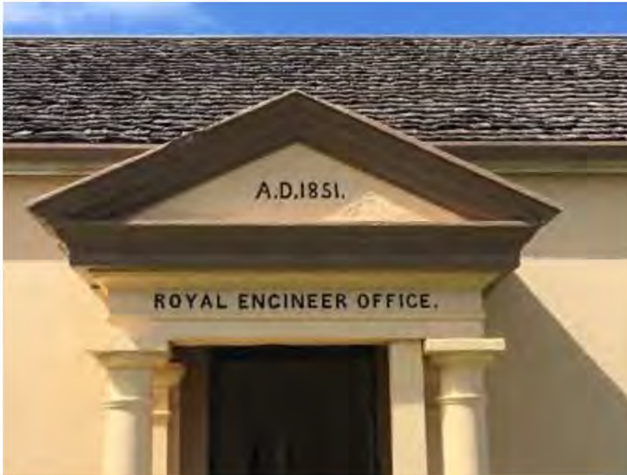
Figure 3 REO Portico Front View
