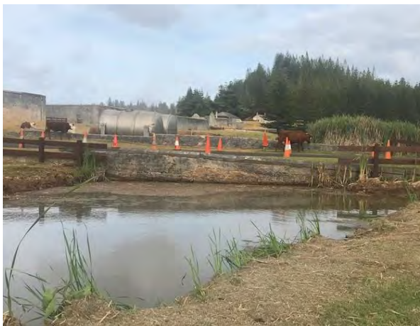
Plate 8 View south-south-west showing eastern wall of the Bounty Street Bridge. Note the patched area where the arch has been amended. AECOM, 2020.
