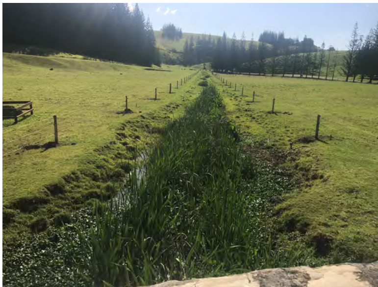
7. main channel to Pier Street showing widening from original interwar photograph
