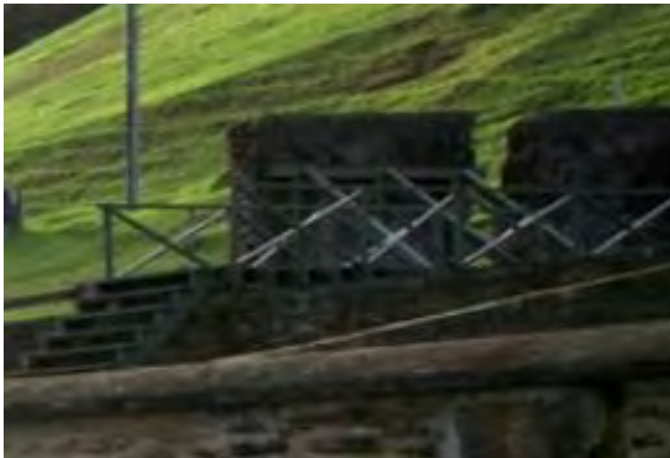
Figure 2 Existing timber braces on Quality Row.
