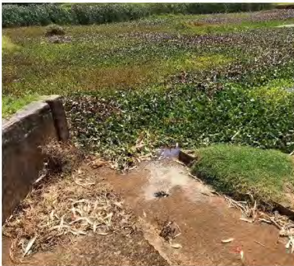
Figure 16 Upstream end of spillway
