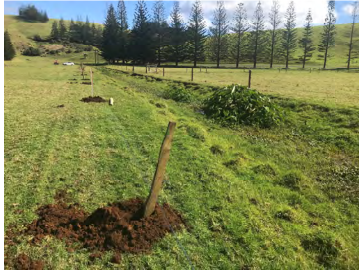
8. Installation of the radially cut traditional posts for the fence.
