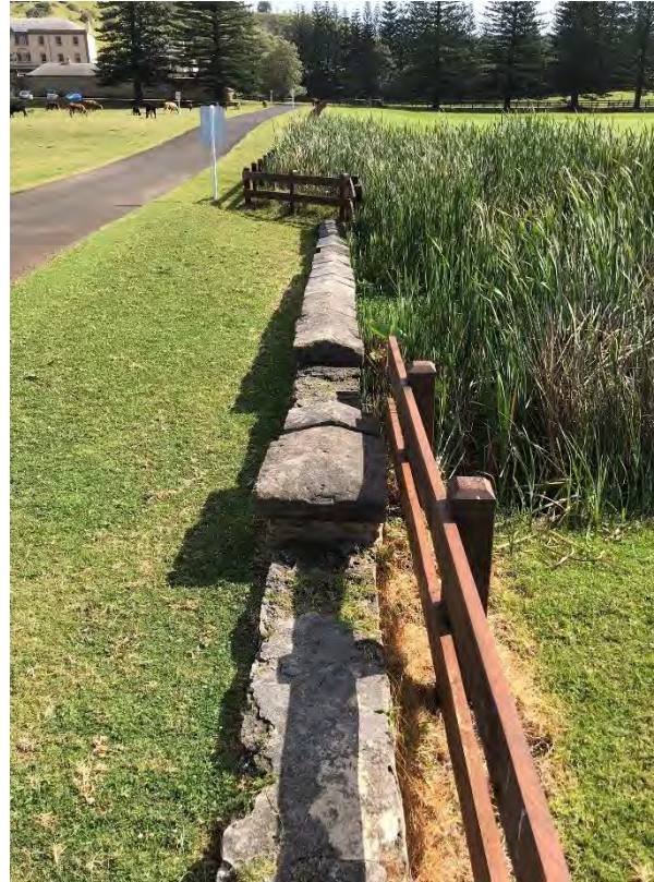
Plate 7 View north along Bounty Street showing eastern wall of Bridge. AECOM, 2020.
