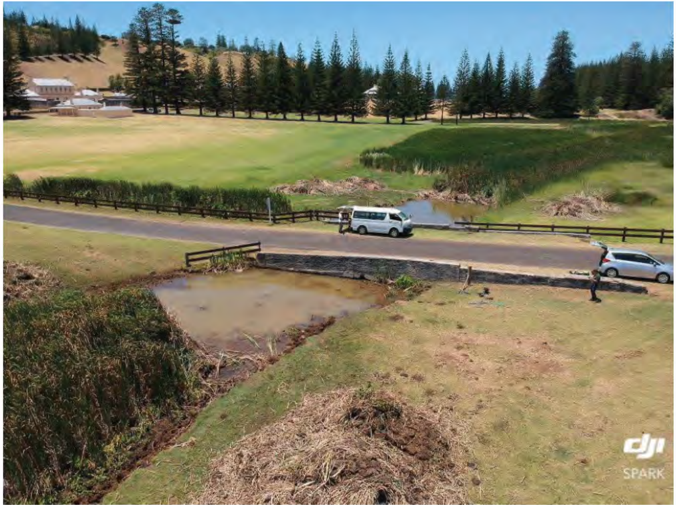
Photo 5 – 28/1/2020 – View of the site looking east.
