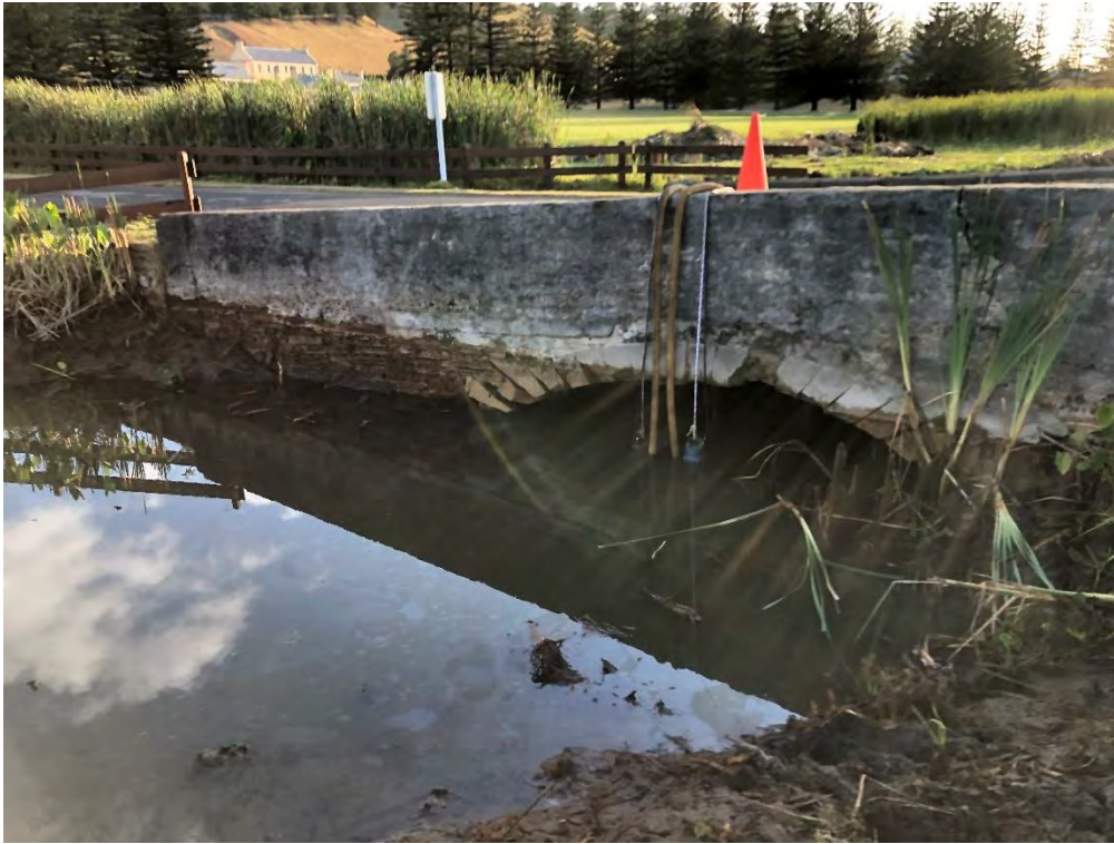
Figure 6 Dewatering Prior to Inspections
