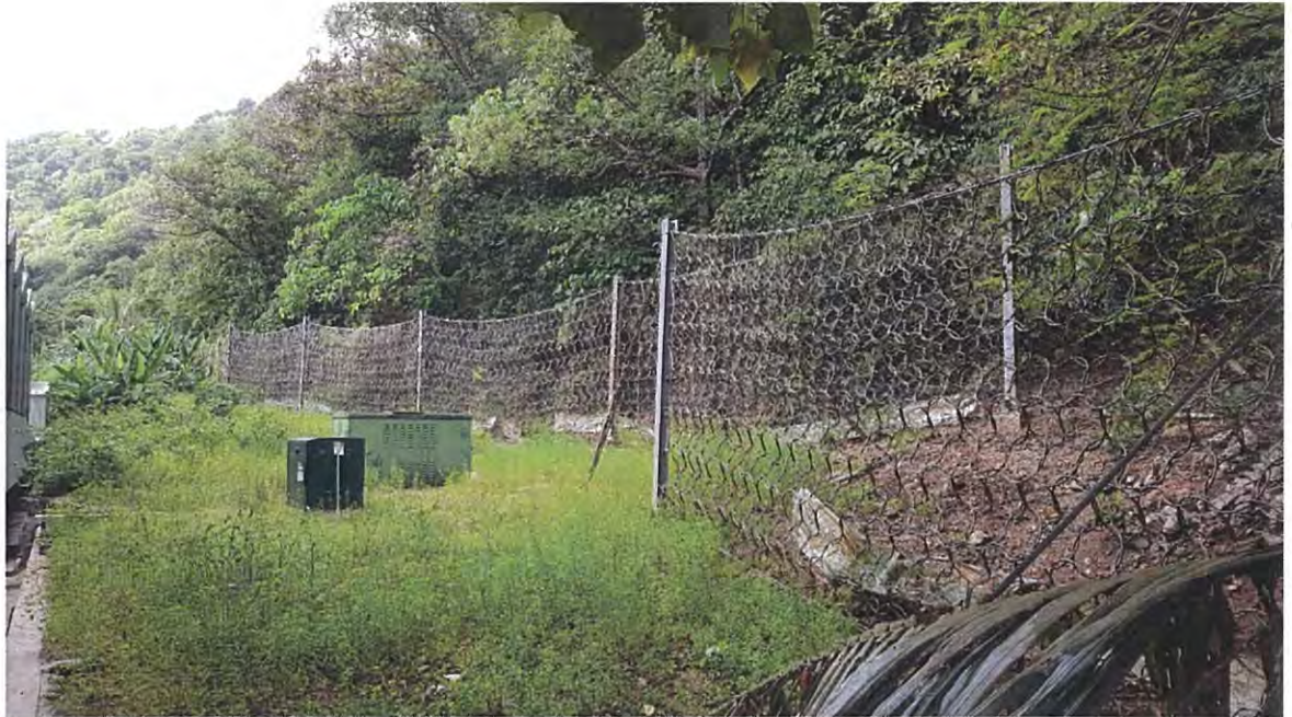
Figure 8. View of Rockfall Barrier behind the Marine 1 building
