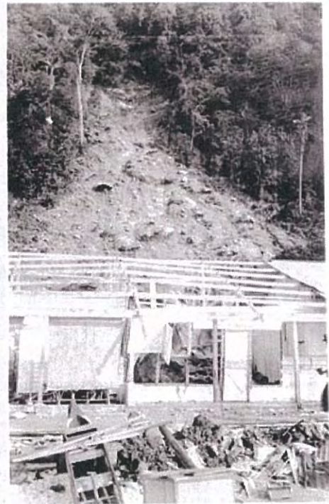
Landslide above the Malay house, from the top of the slide. Note the extent of landslide run out.
