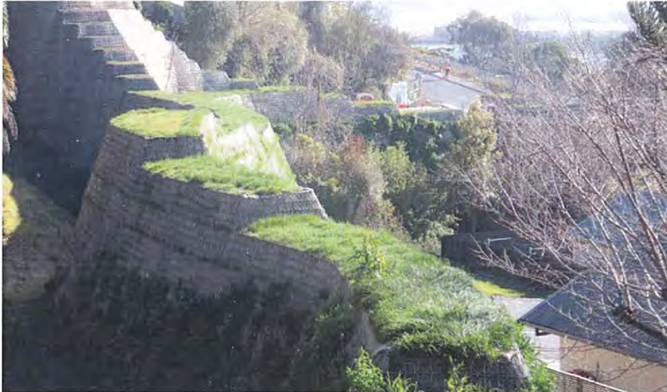
Figure 17. Green Terramesh® embankment providing debris flow protection to residential area, Christchurch, New Zealand. (Photo courtesy of Maccaferri Pty Ltd / Geofabrics)
