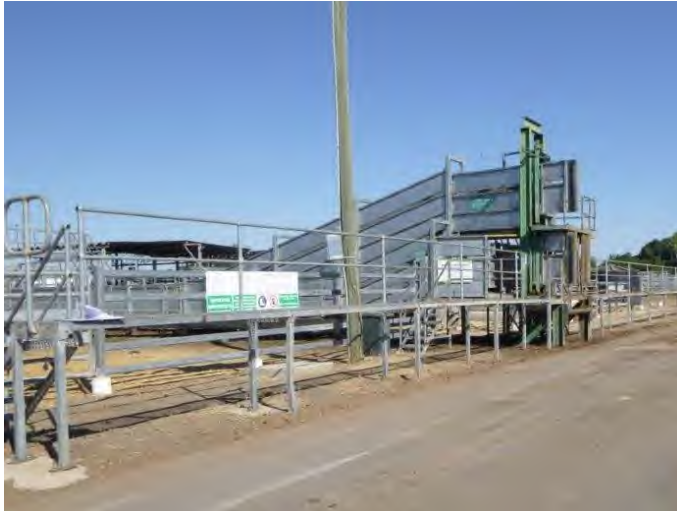
Figure 6: Existing double-decker single width in and out loading ramp.
