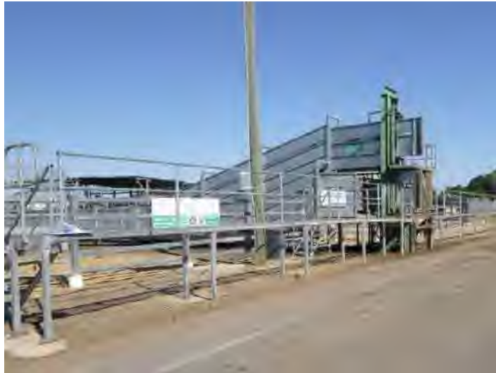
[Figure 5: Existing double-decker single width in and out loading ramp]
