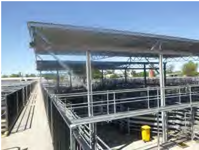
Figure 4: Existing roof structure over draft yard - extended to new roof over Scale-house.
