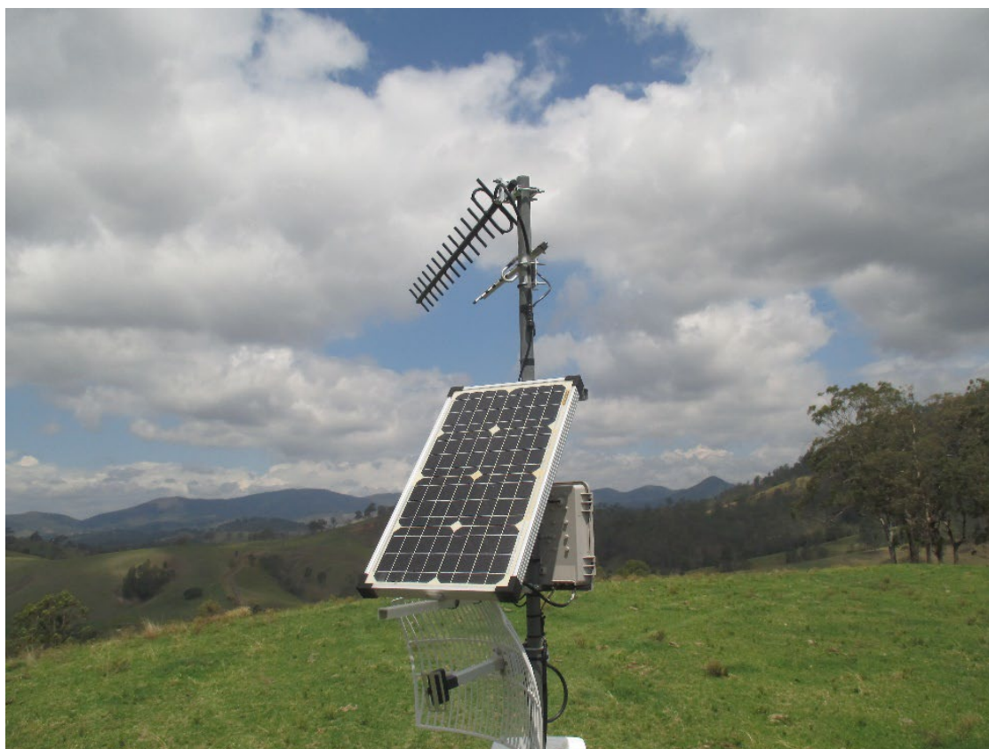
Figure A6: Solar-powered 700 MHz 4G relay, Wahroonga Farm ridge (600 m from homestead; 39 km to Telstra tower). Uninterrupted through both rain events. 700 MHz is rain-transparent at all Australian rainfall intensities.
