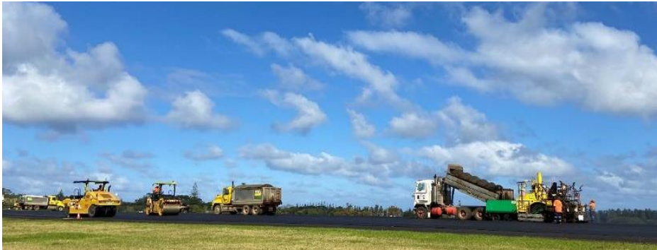
Placement of Asphalt wearing course on Runway 11/29
