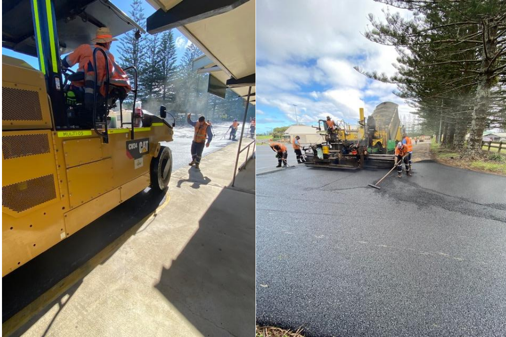
Paver placement of Asphalt wearing course on Airport Car Park
