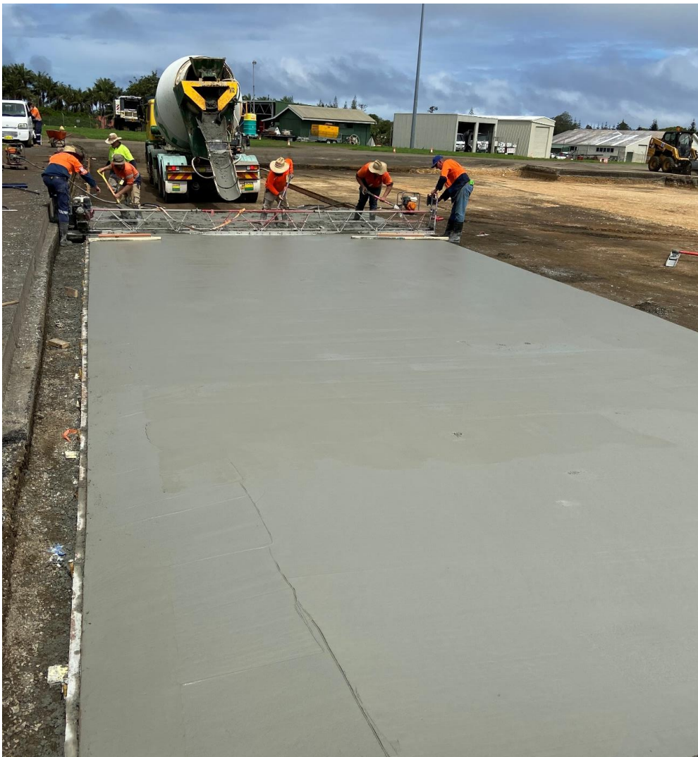
Placement of lean mix layer for RPT Parking Bay 2
