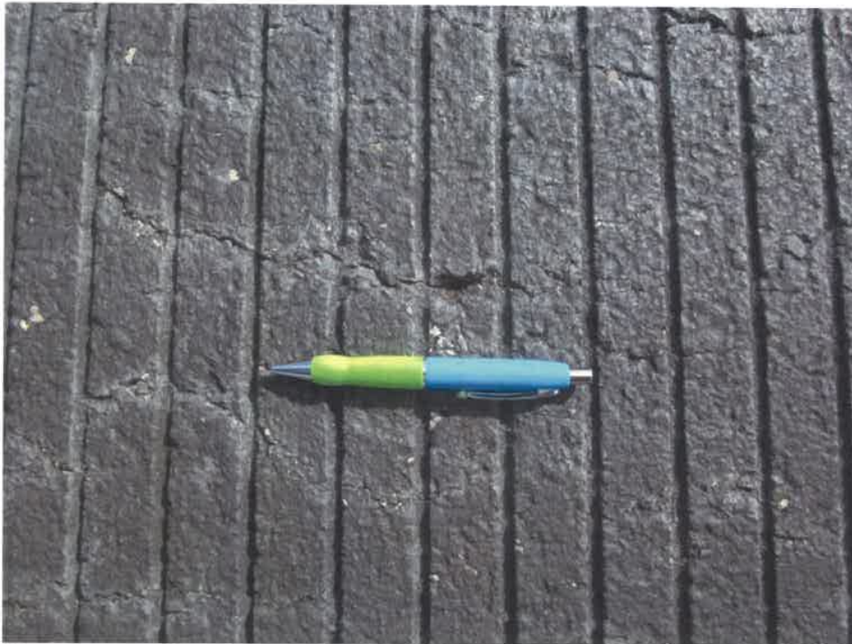
Photo 3. Area of top down cracking treated with bitumen emulsion based product.
