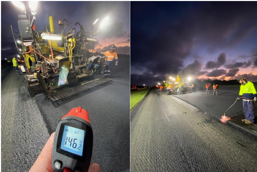
Asphalt wearing course placement
