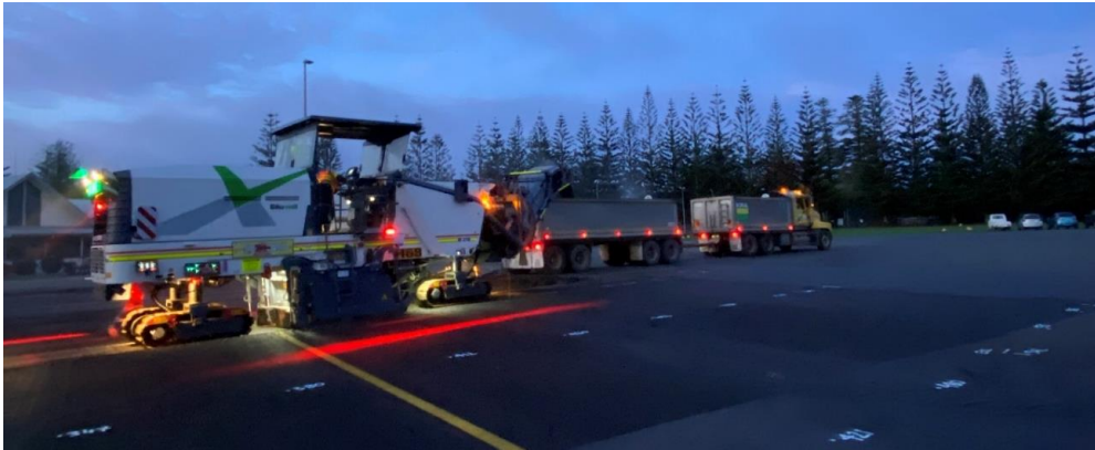
Profiling of concrete pad for Bay 1
