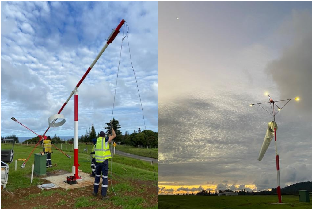
Illuminated Wind Direction Indicator commissioning
