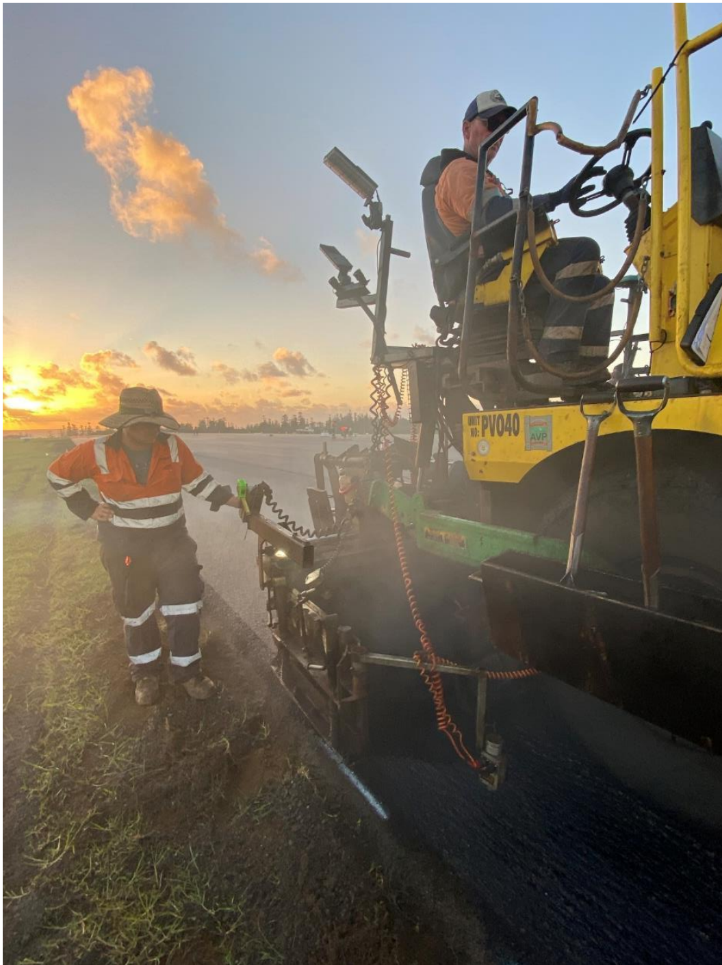
Placement of Asphalt wearing course on Runway 11/29
