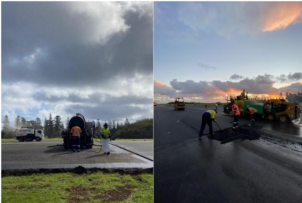
Asphalt wearing course placement
