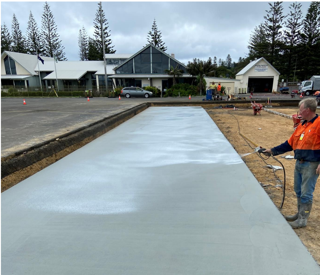
Application of curing membrane on lean mix layer for RPT Parking Bay 2
