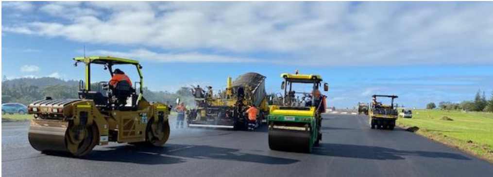
Asphalt wearing course placement
