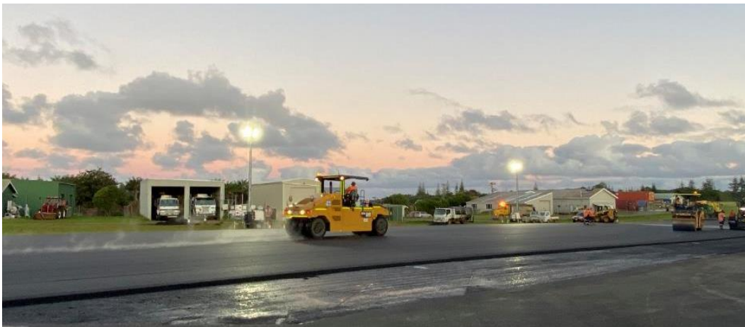
Roller compaction of Taxiway Asphalt wearing course
