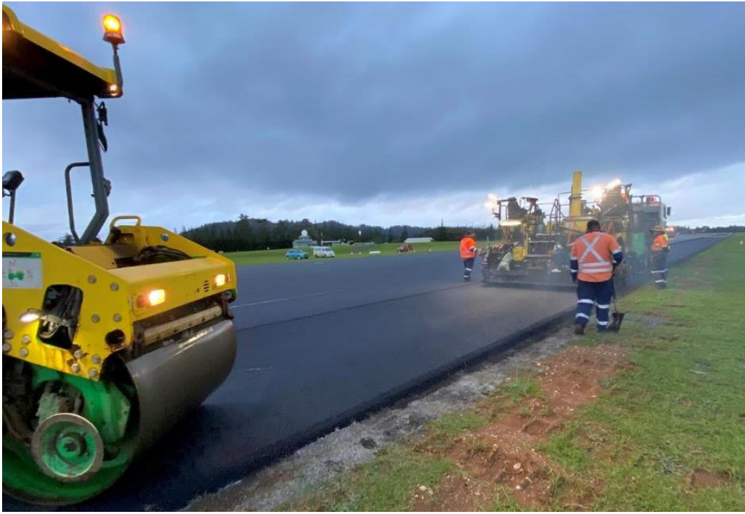
Paver placement of Asphalt wearing course on Runway 04/22
