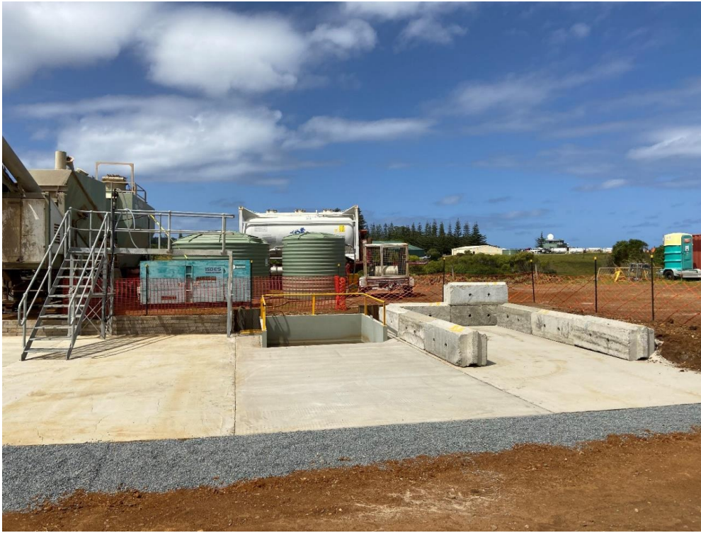
Establishment of Concrete batching plant
