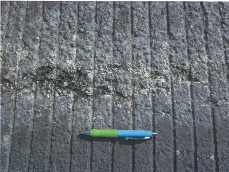
Photo 4. Severe ravelling and erosion of paving run joint.
