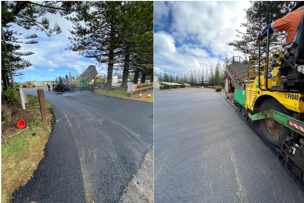
Paver placement of Asphalt wearing course on Airport Car Park
