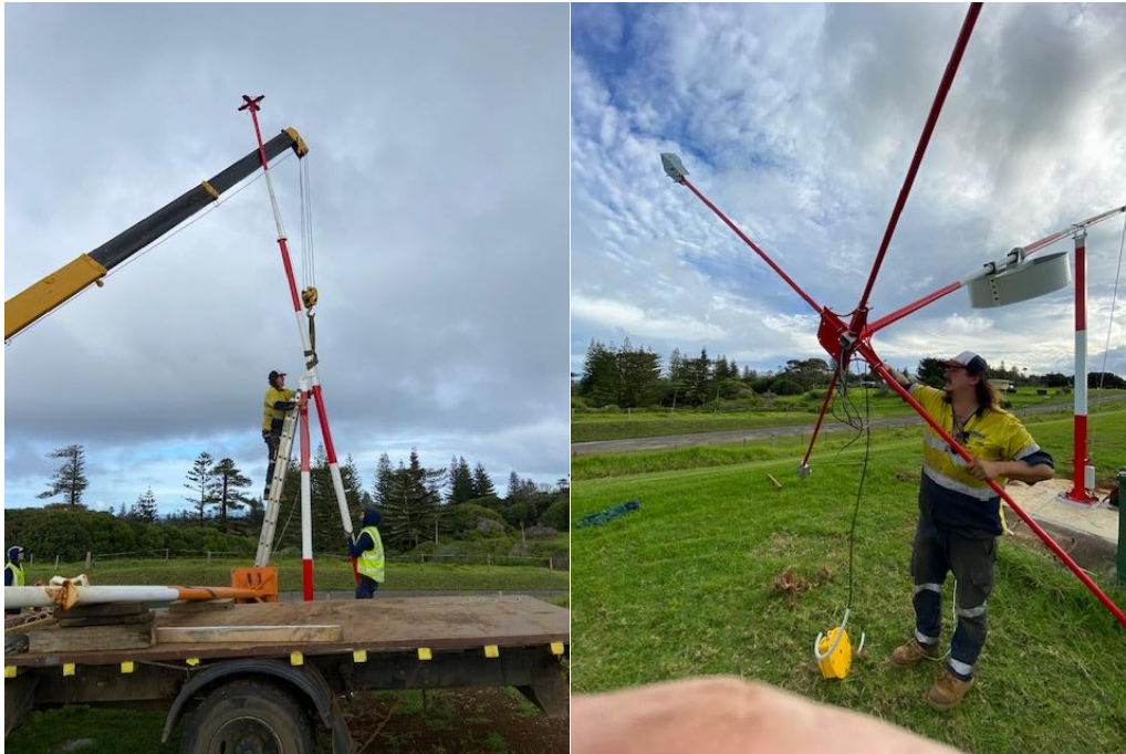
Illuminated Wind Direction Indicator commissioning
