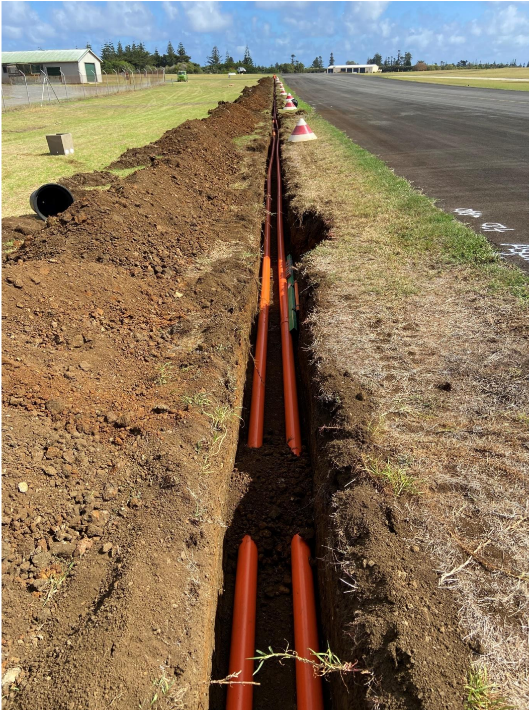
Installation of Airfield Ground lighting twin 80mm conduit along Taxiway
