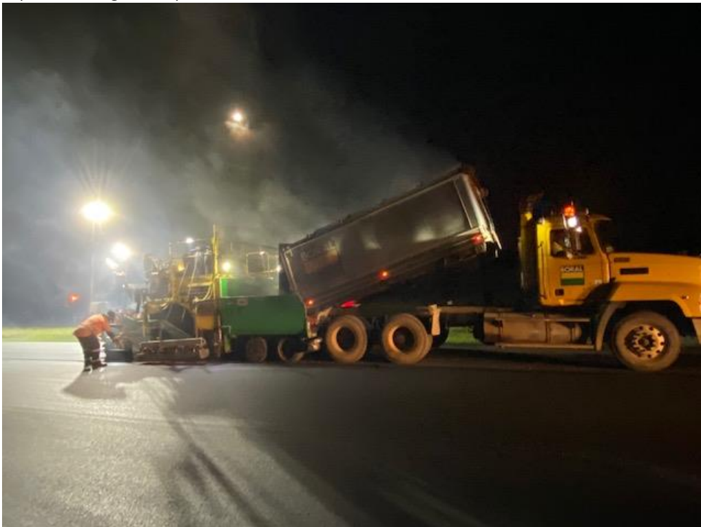
Asphalt wearing course placement
