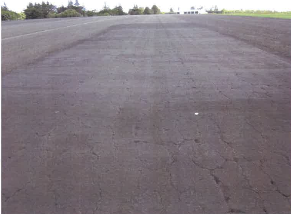
Photo 5. Taxiway rutting with cracking on taxiway, treated with bitumen emulsion based product.
