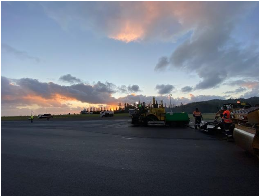
Asphalt wearing course placement
