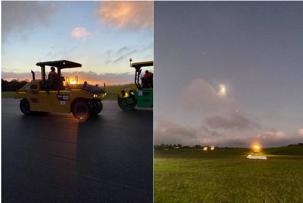
Asphalt wearing course placement
