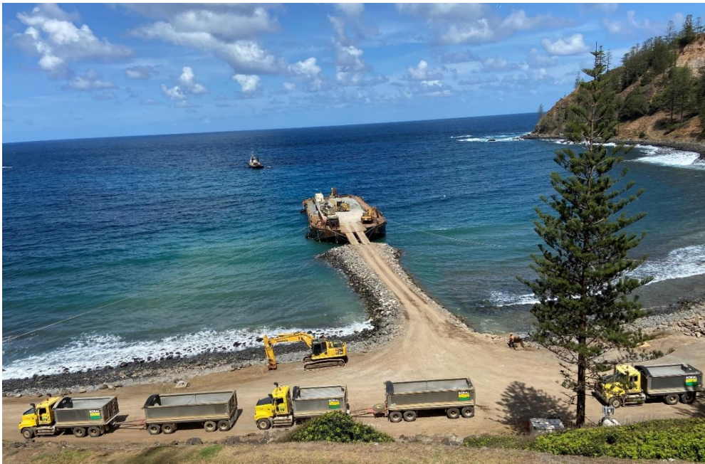
Unloading of aggregates for asphalt and concrete production
