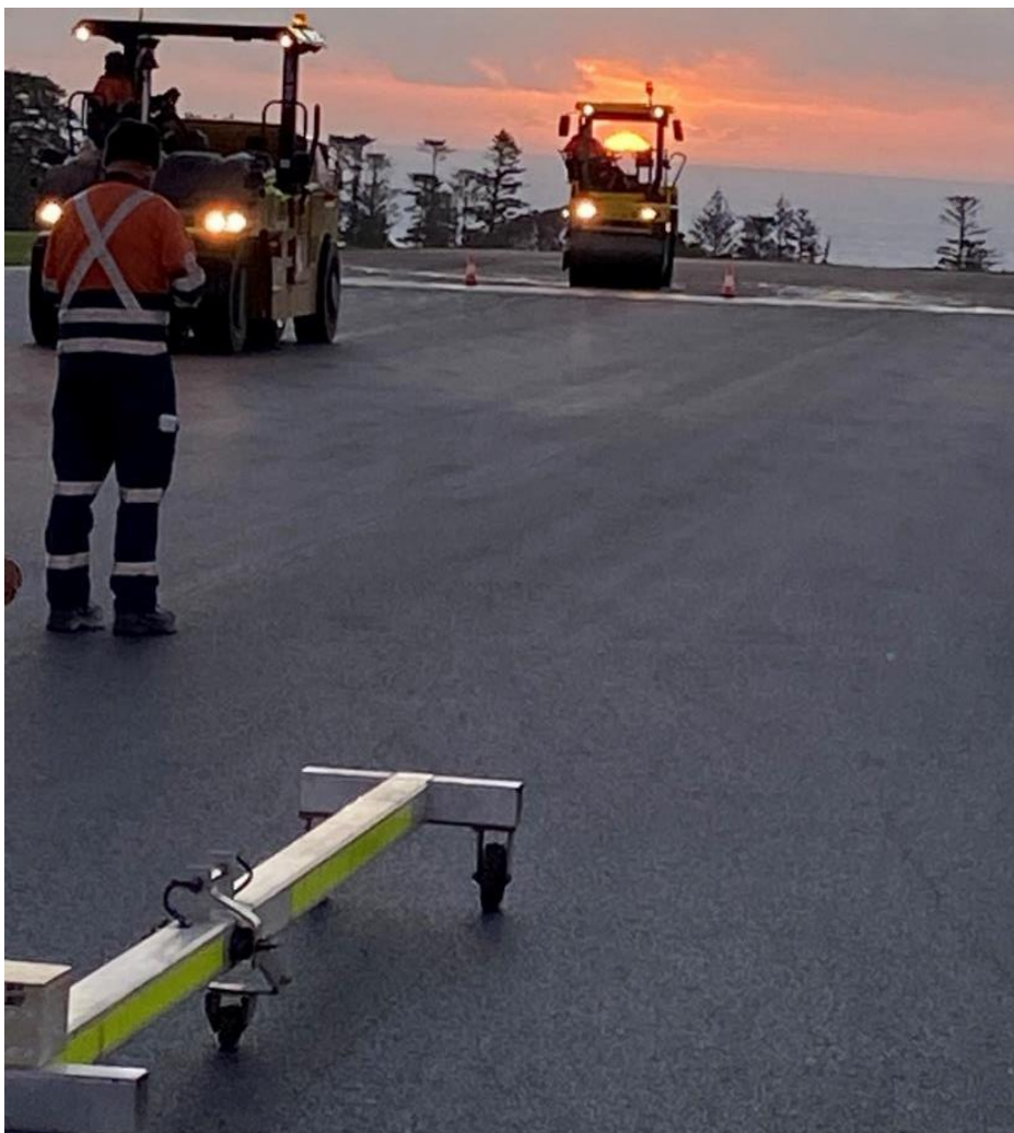
Roller compaction, survey pick up and rolling straight edge testing Runway 11/29 Asphalt wearing course
