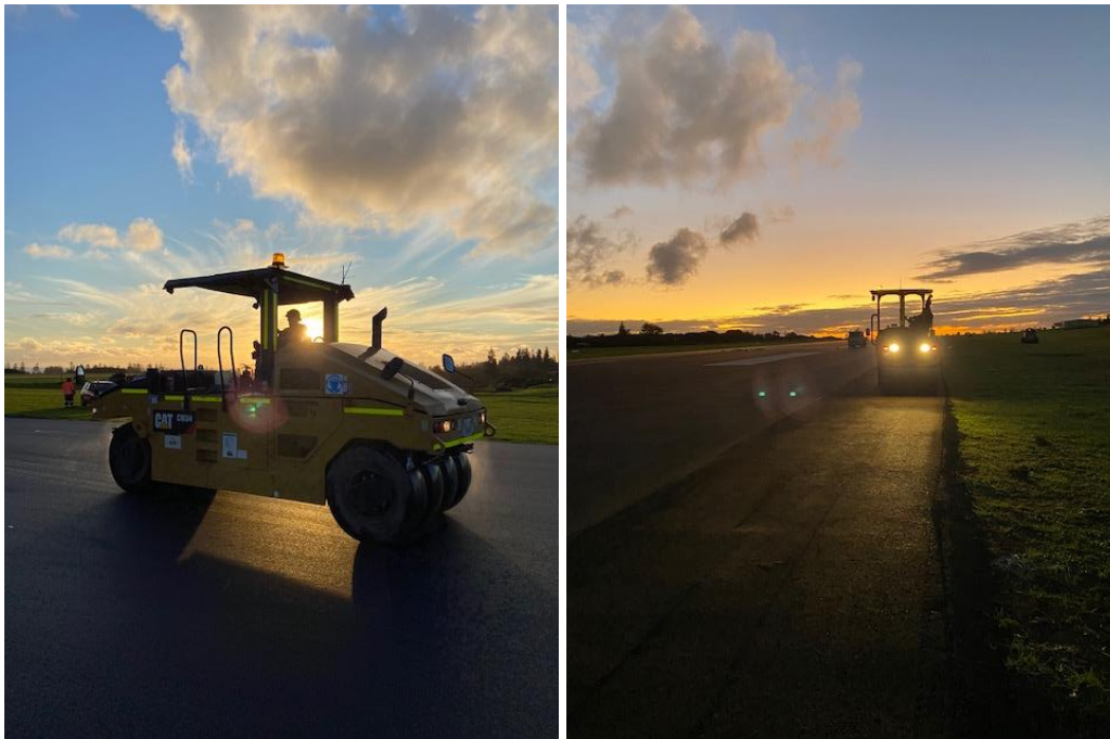
Asphalt wearing course placement
