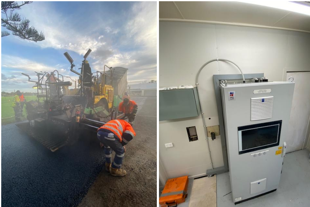
Asphalt wearing course placement
