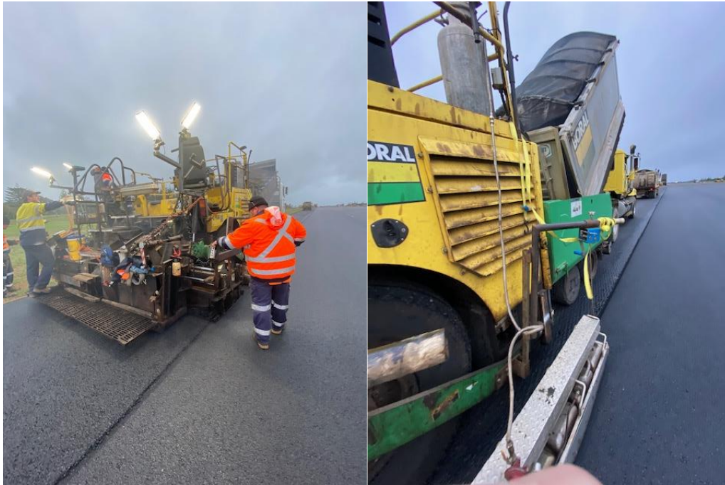
Asphalt wearing course placement
