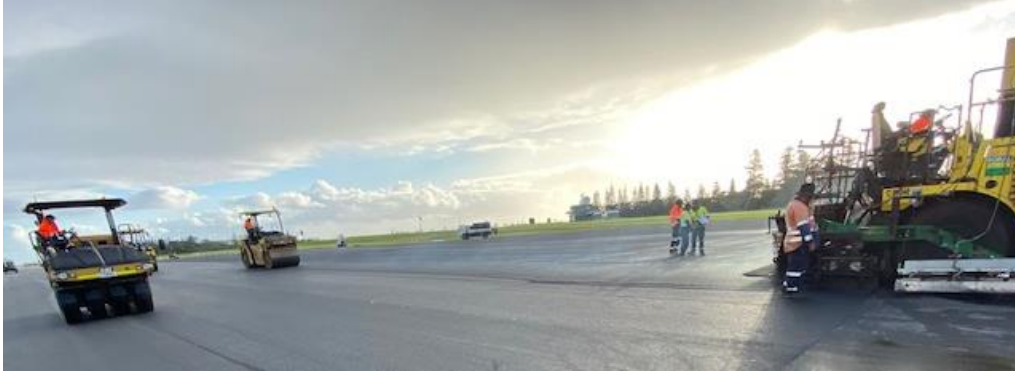
Asphalt wearing course placement
