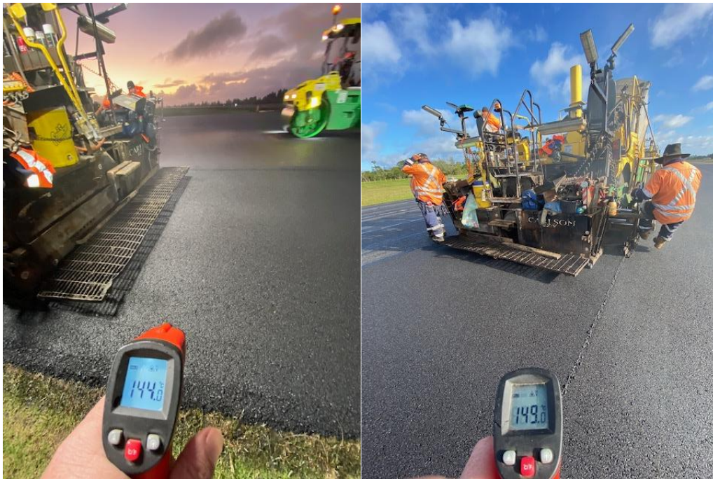
Asphalt wearing course placement
