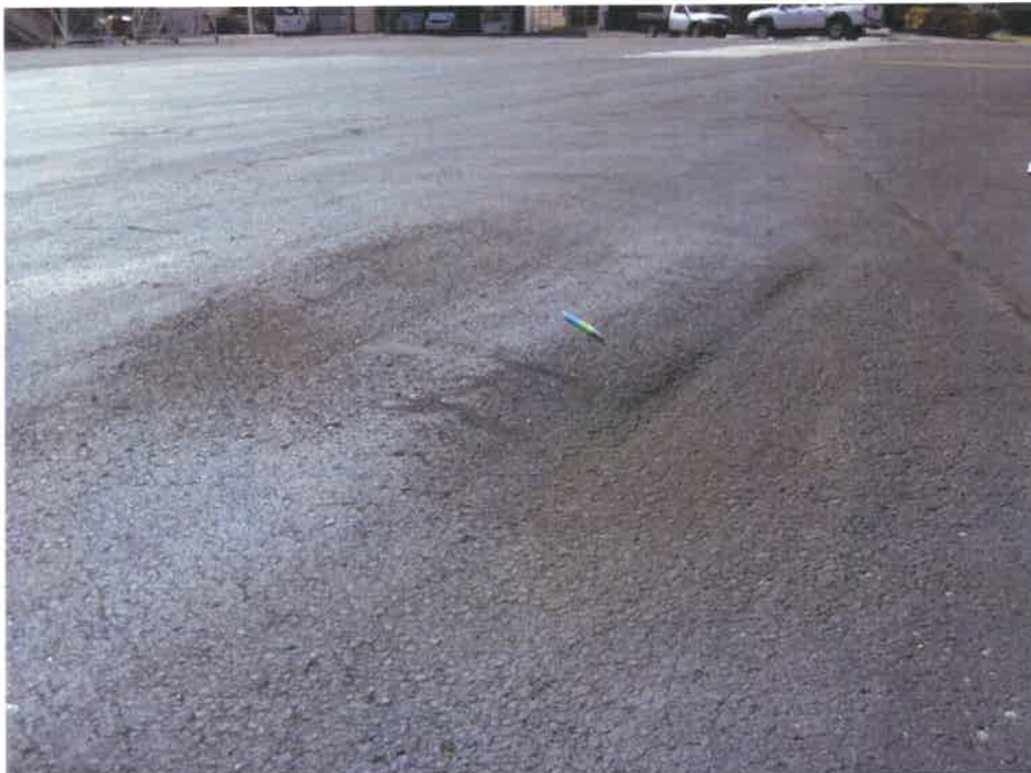
Photo 6. Severe asphalt deformation on parking apron Bay 1.
