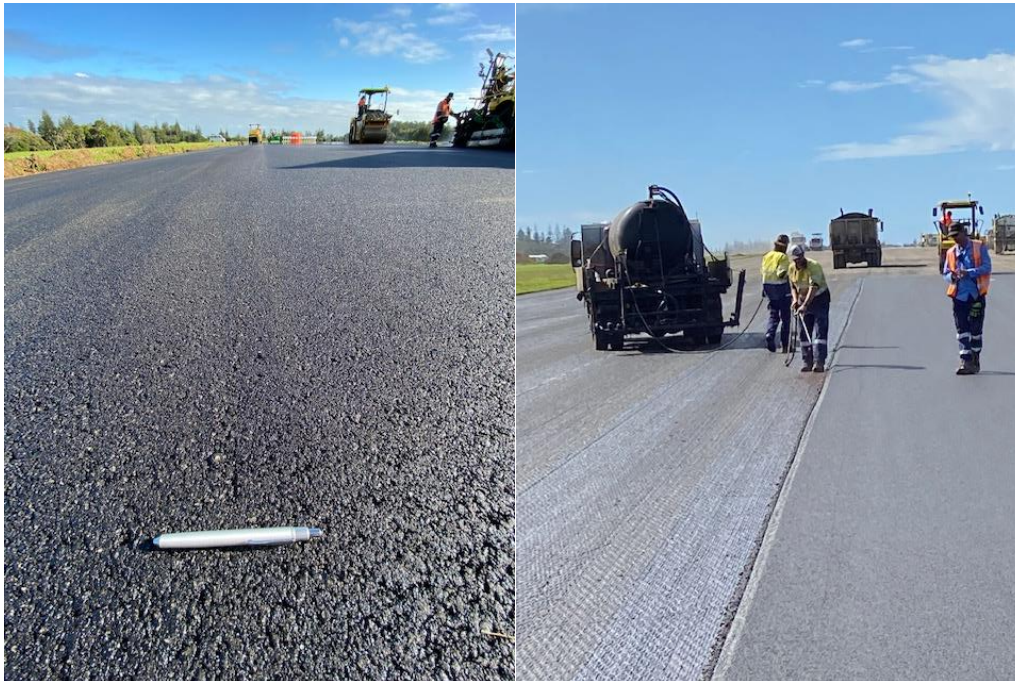
Asphalt wearing course placement
