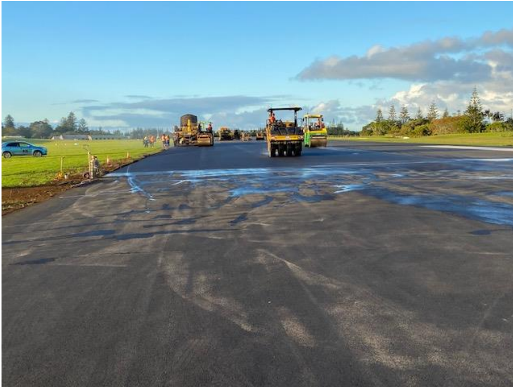
Asphalt wearing course placement
