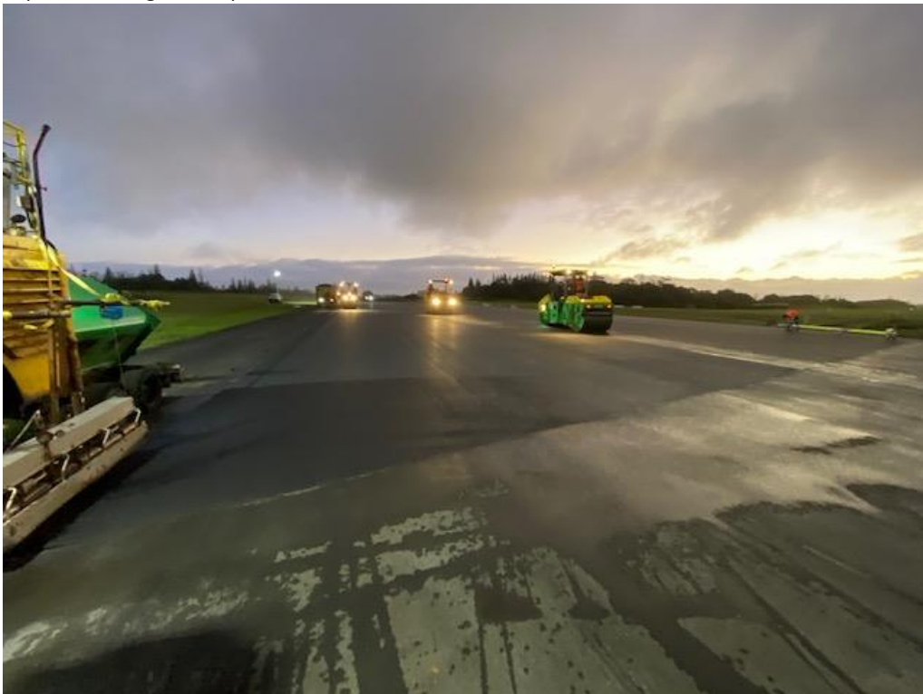
Asphalt wearing course placement
