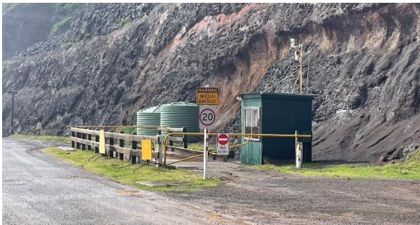
PHOTOGRAPH 2-5 WATER TANKS AND WEIGHBRIDGE (ERM 2025)
