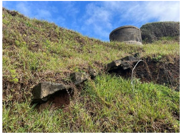
PHOTOGRAPH 2-14 UPPER PLATFORM WITH CONCRETE TANK AND STAIRS (ERM 2025)
