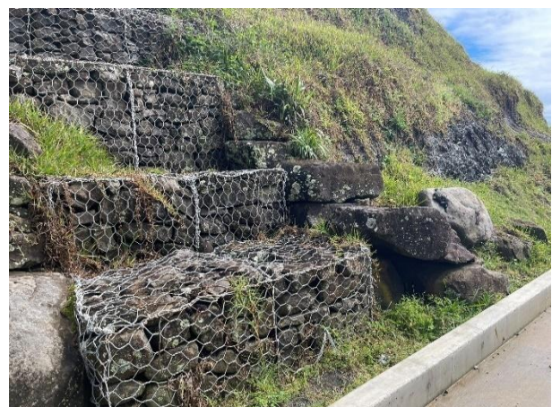
PHOTOGRAPH 2-12 UPPER PLATFORM WITH SLOPE STABILISATION (ERM 2025)
