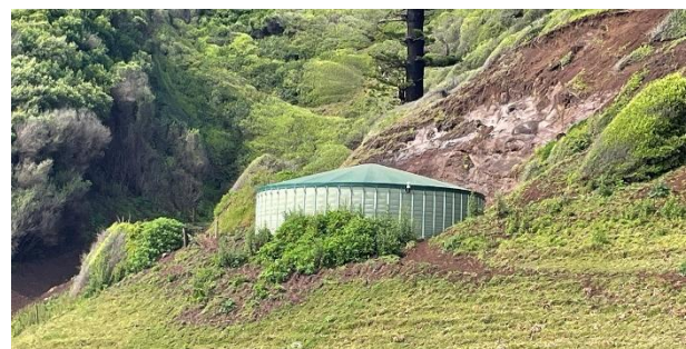
PHOTOGRAPH 2-8 DESALINATION PLANT WATER RESERVOIR (ERM 2025)
