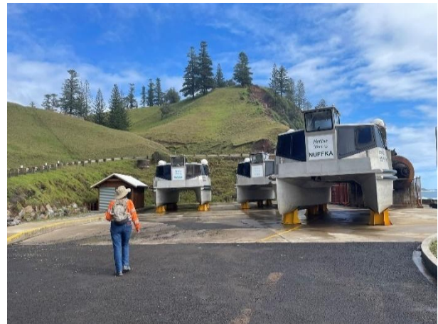
PHOTOGRAPH 2-10 UPPER PLATFORM WITH RESURFACING, KERBING, PUBLIC TOILET (ERM 2025)
