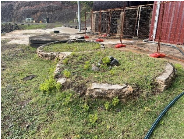
PHOTOGRAPH 2-13 UPPER PLATFORM WITH FORMER CONCRETE TANKS (ERM 2025)
