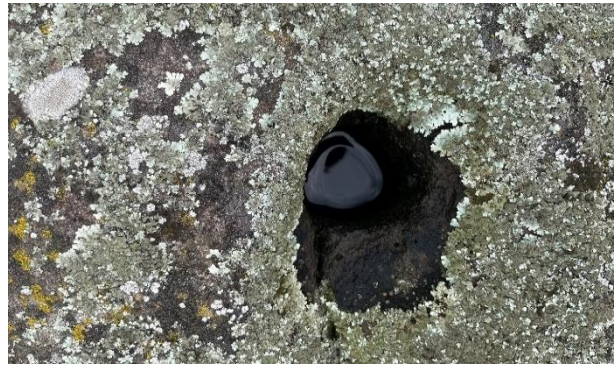
PHOTOGRAPH 2-24 POTENTIAL SURVEY POLE HOLE (ERM 2025)
