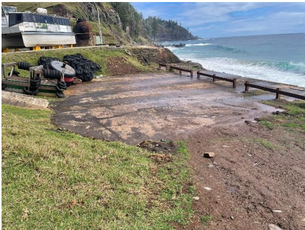
PHOTOGRAPH 2-9 LOWER PLATFORM WITH RAMP AND STAIRS (ERM 2025)
