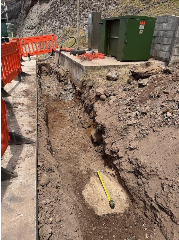
PHOTOGRAPH 5-1 CALCARENITE SLAB IN DESALINATION PLANT TRENCH (DITRDCA)
