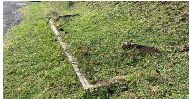
PHOTOGRAPH 2-6 CONCRETE REMNANT OF FORMER BUILDINGS (ERM 2025)
