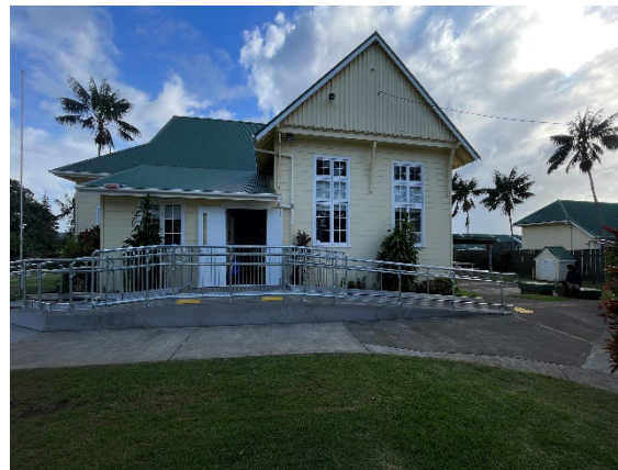
Building D – Accessibility Ramp
