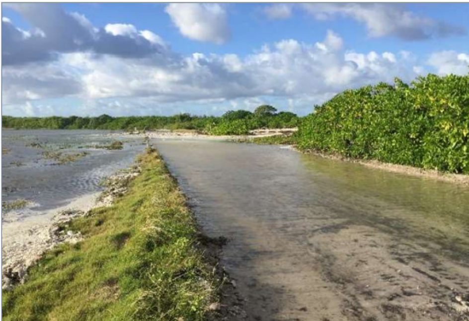
Figure 16: Airforce Road flooding during July 2018 storm event (RHDHV, 2021a – source: David McKinney)
