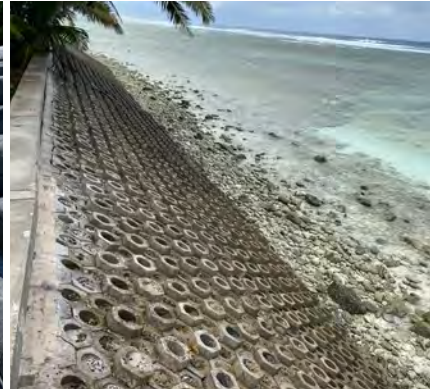
MU1: West Island Settlement - Seabee seawall
