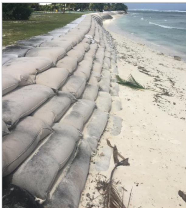
Figure 21: Photo of William Keeling GSC seawall as an example of a typical GSC seawall (RHDHV 2021b)
