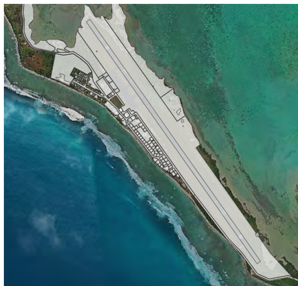
Figure 57: West Island whole of settlement
