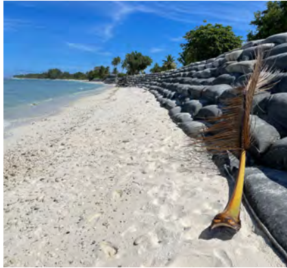
MU1: West Island Settlement - GSC sandbag seawall
