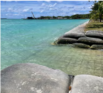
MU 7: Home Island Settlement - Jalan Pantai seawall
