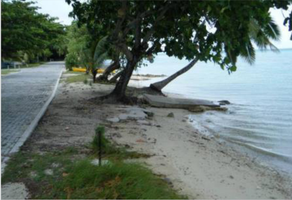
Figure 11: Jalan Pantai on Home Island prior to seawall construction (1) indicating the low elevation of the road and narrow foreshore, 29 May 2009 (DoT, 2010)
