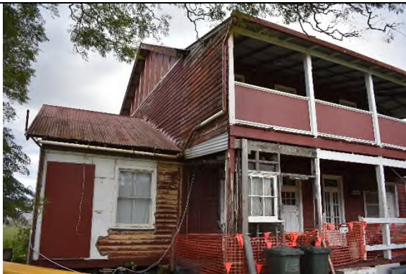
Figure 133 Southeastern corner of Christian's Minde. Exposed weatherboard on left and inset window in verandah are the location of a removed annexe.
