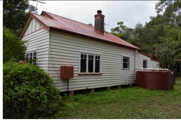
Figure 85 Southern elevation of Pamir Cottage.
