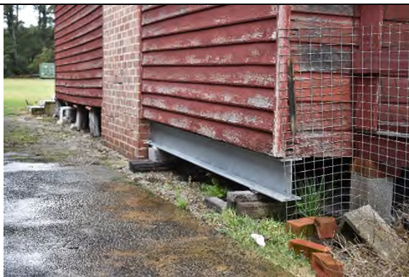
Figure 141 Steel beam inserted to provide structural support to foundations.
