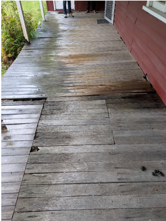
Figure 115 Patched sections of verandah boards.
