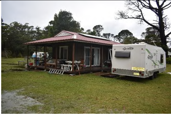
Figure 16 E2, viewed from northwest.
