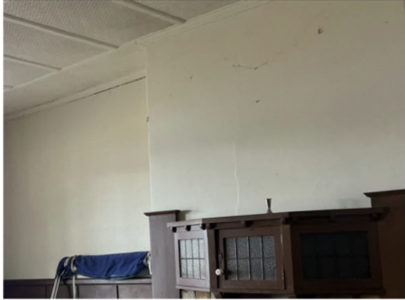
Figure 147 Ground floor interior, 2024, showing potentially significant cabinetry. (Source: ACOR Block 14 Building Audit Report)
