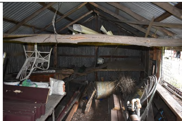
Figure 81 Interior of Pop's Shed.
