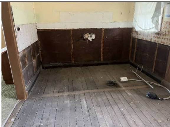
Figure 145 Ground floor interior, 2024. (Source: ACOR Block 14 Building Audit Report)
