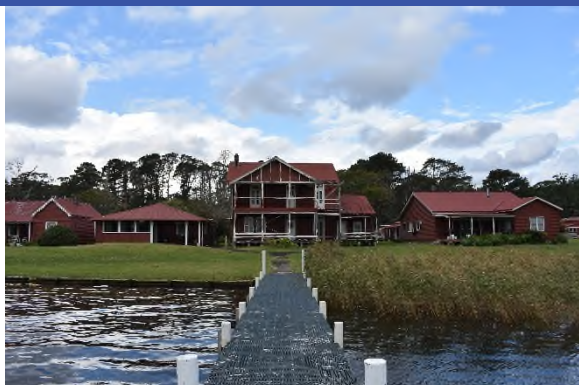
Figure 127 CM3 (Christian's Minde) at centre of image viewed from jetty, with CM2 and CM1 to the left, and CM11 to the right.
