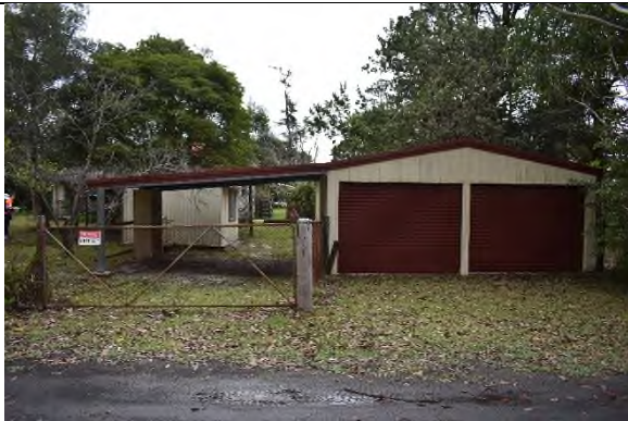
Figure 98 Garage and other outbuildings.
