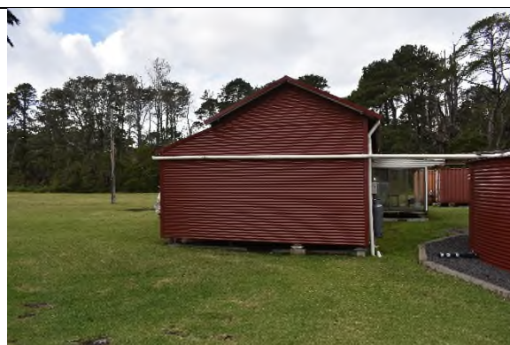
Figure 156 Western elevation of CM5.
