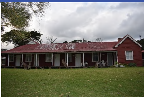
Figure 101 Western elevation of CM1.
