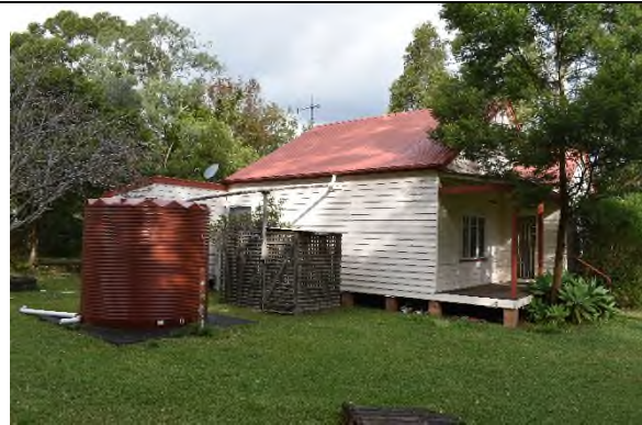
Figure 87 Northwestern corner of Pamir Cottage, showing main entrance and verandah.
