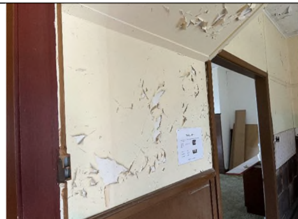
Figure 146 Ground floor interior, 2024. (Source: ACOR Block 14 Building Audit Report)
