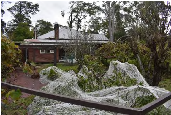
Figure 70 Eastern elevation of A1 (Ardath Cottage).
