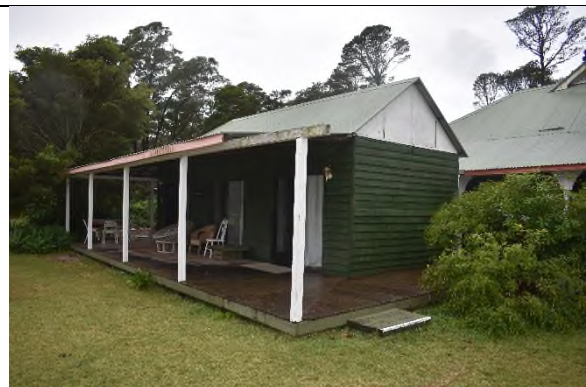
Figure 48 Northern annexe with unfinished verandah frame.
