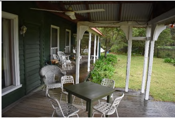
Figure 25 Southwestern verandah, K1.
