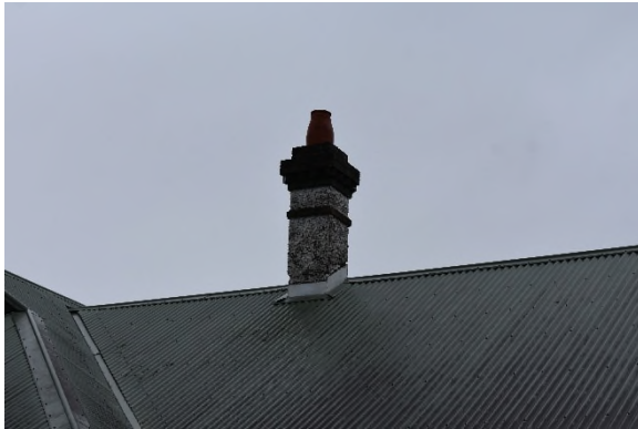
Figure 43 Detail of chimney.
