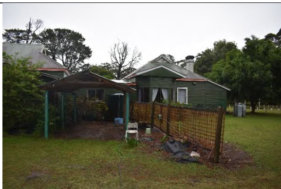
Figure 29 Southern elevation, showing eastern annexe on right, K1.
