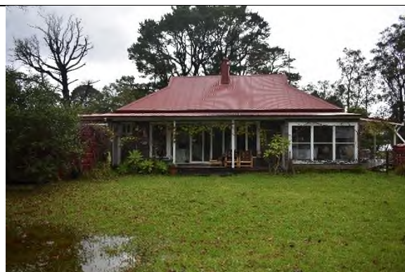
Figure 7 Western elevation of E1.
