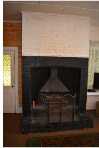
Figure 38 Fireplace in accommodation areas in K1.
