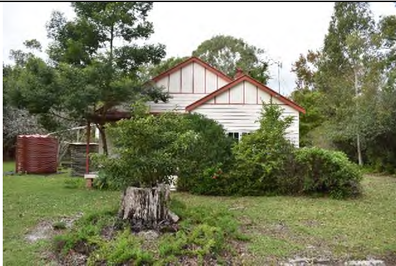
Figure 86 Western elevation of Pamir Cottage.
