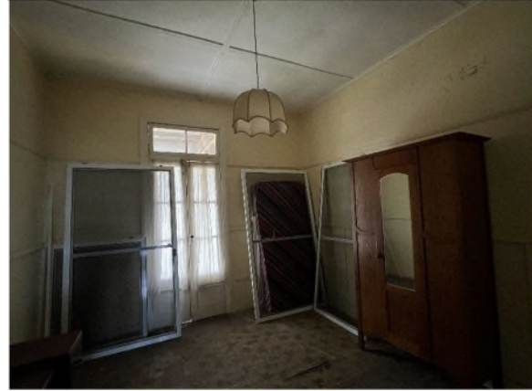
Figure 148 Ground floor interior, 2024. (Source: ACOR Block 14 Building Audit Report)
