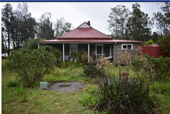
Figure 2 Eastern elevation of E1.
