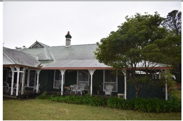
Figure 26 Southwestern verandah, K1.
