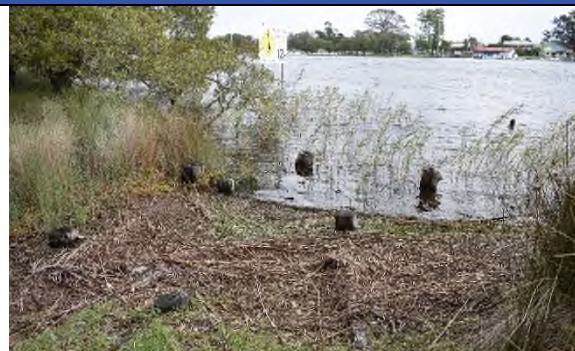
Figure 161 CM7, remnants of the boathouse footings.
