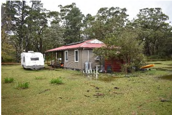
Figure 14 E2, viewed from southeastern corner.
