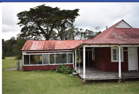
Figure 102 Northern end of western elevation, showing cardroom.
