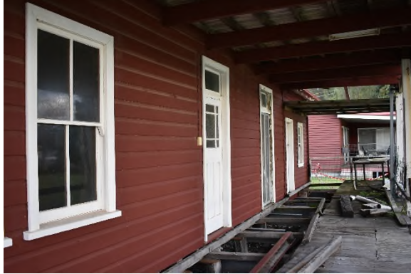
Figure 139 Western verandah, with removed floorboard to provide access to subfloor space.
