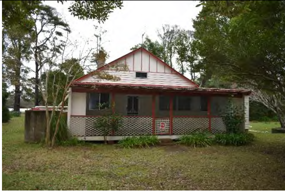
Figure 84 Eastern elevation of P1 (Pamir Cottage).
