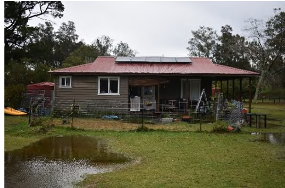
Figure 15 Eastern elevation of E2.
