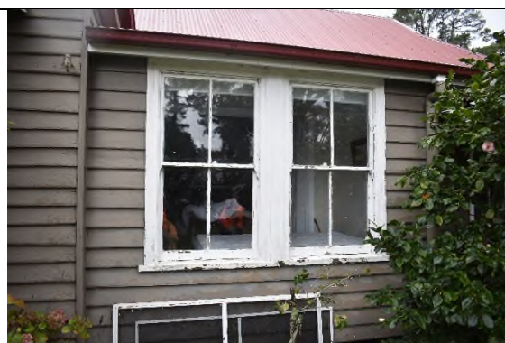
Figure 5 Detail of original timber-framed windows of E1.
