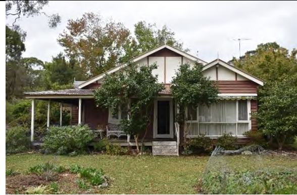
Figure 73 Western elevation of Ardath Cottage.
