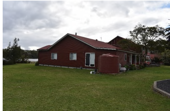
Figure 169 CM11 viewed from south.
