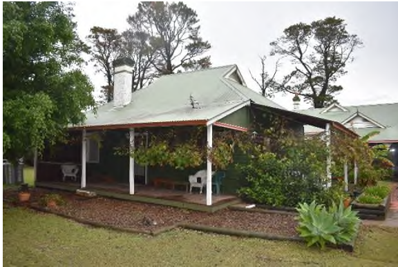
Figure 31 Northeastern elevation showing eastern annexe, K1.
