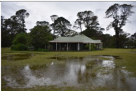
Figure 35 Northern elevation, looking at the northern annexe of K1.
