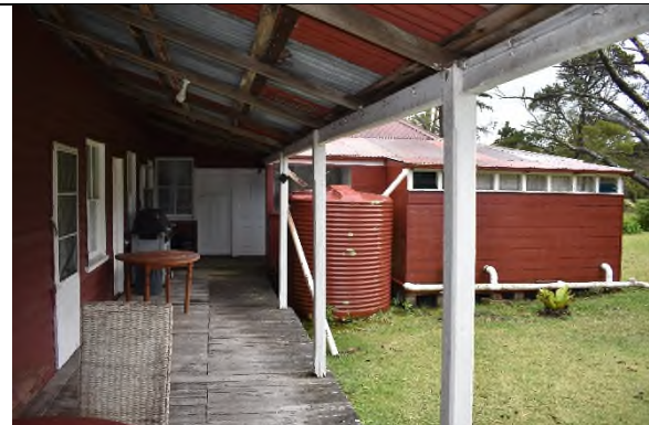
Figure 108 Eastern elevation, with ablutions block on the right.
