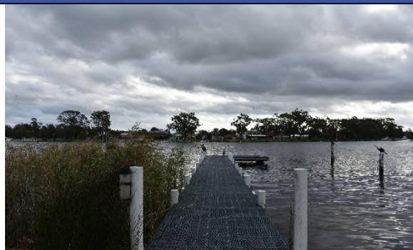
Figure 160 CM6—Block 14 jetty, looking towards Sussex Inlet.
