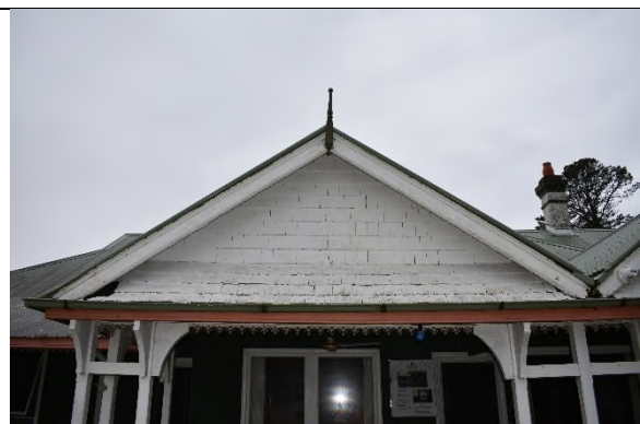
Figure 42 Shingled gable end, southwestern elevation.
