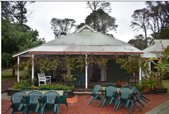
Figure 33 BBQ area, looking south at eastern elevation's northern side.
