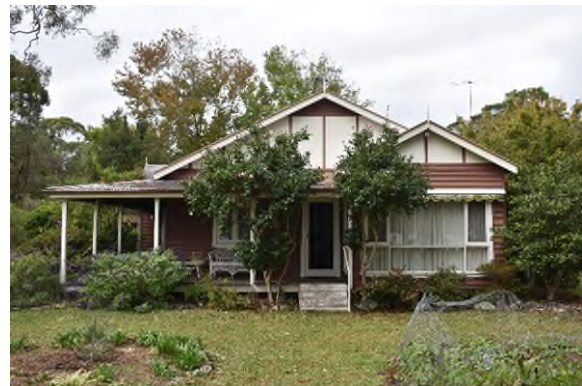
Figure 3.57 The western elevation of Ardath Cottage (Building A1).
