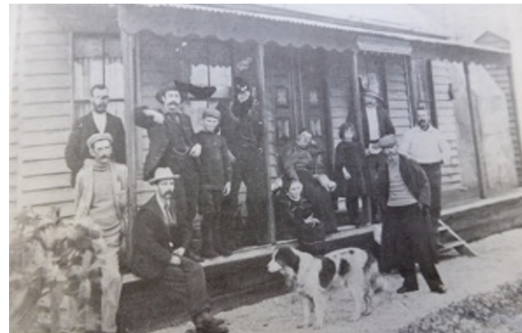
Figure 2.11 Ellmoos family and guests at Christian's Minde in the early days. Date unknown. Note the symbols on the front door of the main cottage—a Danish custom—and the name on the front porch over the steps. (Source: Department of the Capital Territory Collection, reproduced from CDHS Journal , March 1981)
