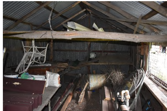
Figure 3.63 The interior of Pop's Shed (Building A3), showing the bush pole framing and simplistic construction.
