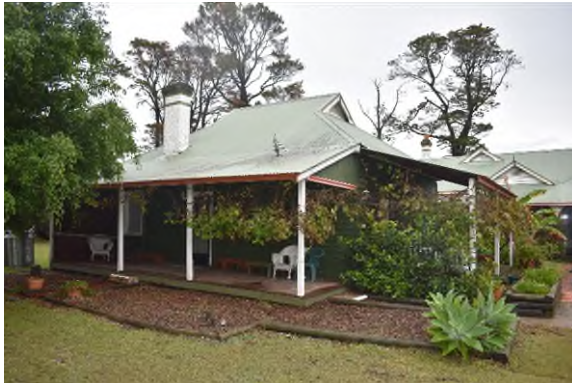
Figure 3.43 The eastern annexe of Kullindi (Building K1).
