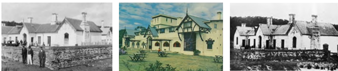
Figures 1–3 The Seahorse Inn in various stages of its construction and evolution. (Source: Eden Community Site, via website < http://www.eden.nsw.au >)
