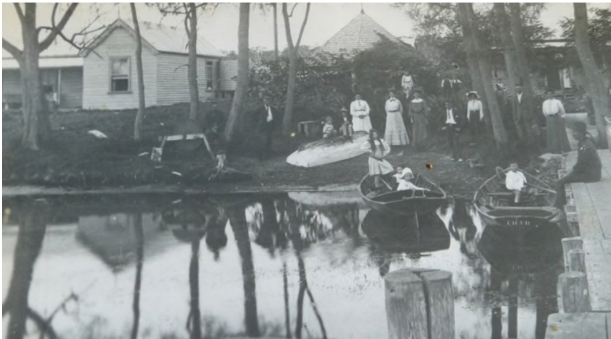
Figure 2.8 Christian's Minde, 1898. The main house is positioned opposite the end of the jetty with the octagonal roofed dining room next door and guest accommodation rooms in the larger cottage along the shore. (Source: Peter and Pam Ellmoos collection)
