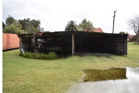
Figure 3.101 The open eastern elevation of the garage and shed, Building CM9.
