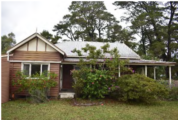
Figure 3.58 The northern elevation of Ardath Cottage (Building A1).
