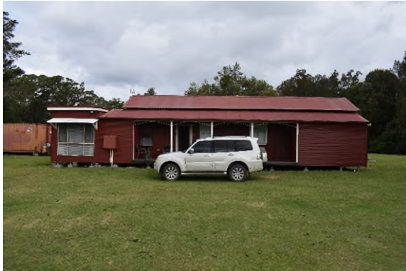
Figure 3.90 The northern elevation of Building CM5—the Staff Quarters.
