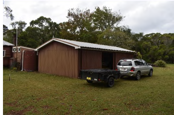
Figure 3.61 Building A2, the c1980s double garage.
