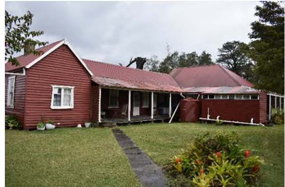
Figure 3.75 The rear (eastern) elevation of Building CM1.
