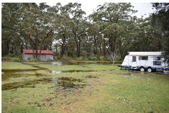
Figure 3.38 Building E3 and the back lawn area, showing the poor drainage at the site.
