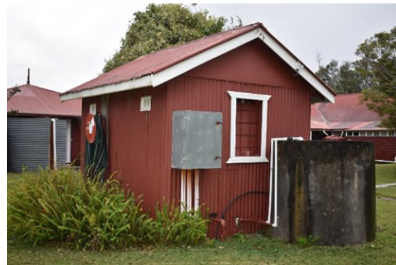
Figure 3.99 The eastern elevation of Building CM8.
