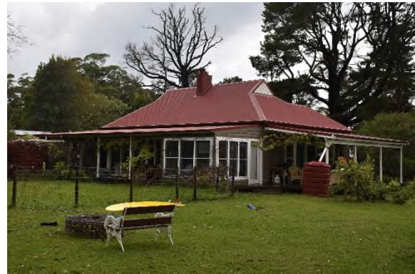
Figure 3.33 Building E1 from the northwest.
