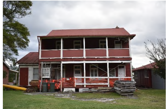
Figure 3.85 The rear (eastern) elevation of Building CM3.
