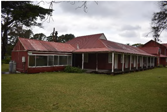
Figure 3.76 Building CM1, with the games/Pontey room on the left of the image.
