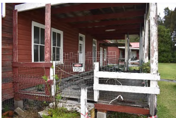
Figure 3.88 The front verandah of Building CM3.
