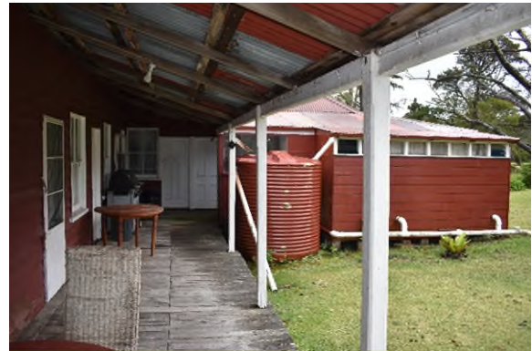
Figure 3.77 The rear verandah of Building CM1, showing the external toilets joined to the building.
