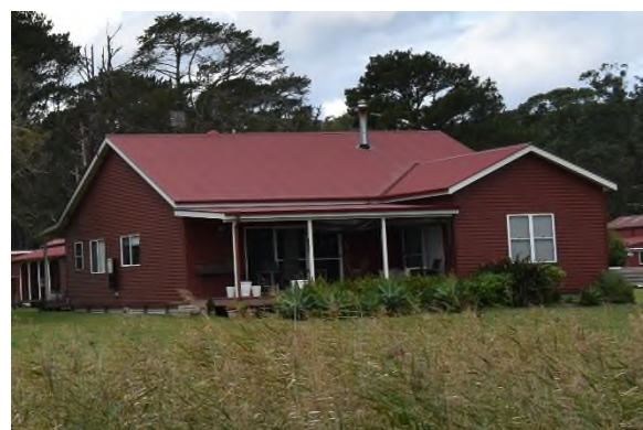
Figure 3.106 The front (western) elevation of Building CM11.
