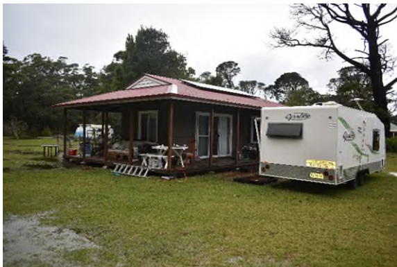
Figure 3.34 Building E2, the c1967 cottage.
