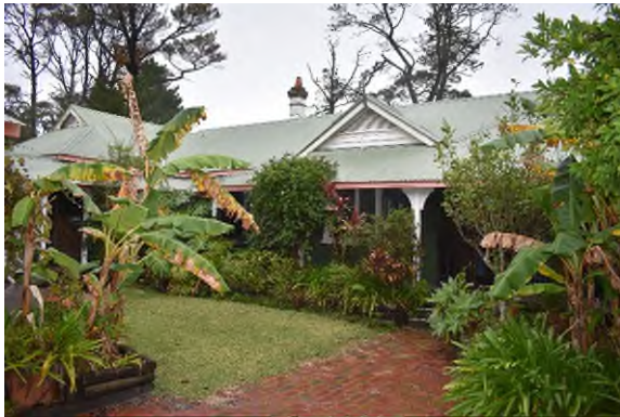
Figure 3.45 The internal courtyard of Kullindi (Building K1), showing the rear of the original homestead building.
