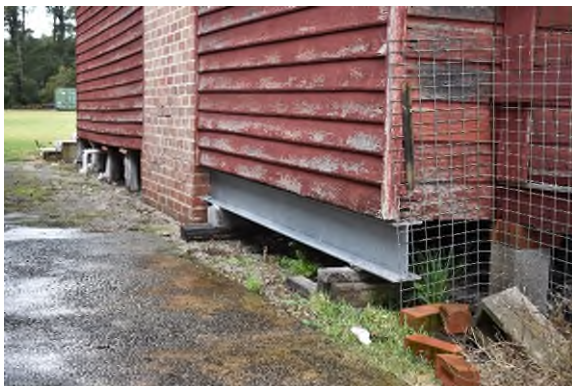
Figure 3.86 Detail of the steel members inserted to shore up the structure of Building CM3.
