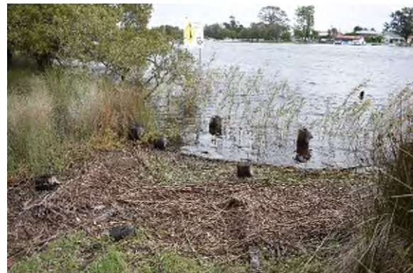
Figure 3.97 The remaining timber stumps of the boathouse—structure CM7.
