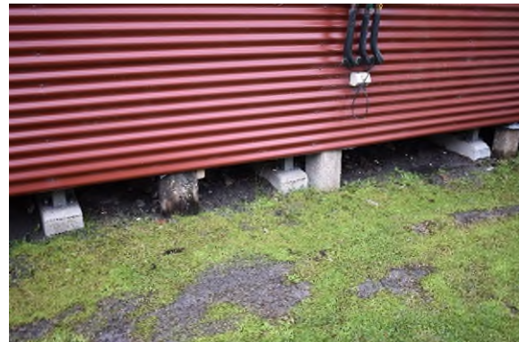
Figure 3.93 New structural footings of Building CM5, using jacks on concrete sleepers.
