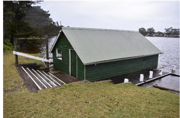
Figure 3.50 The Kullindi Boatshed (Building K2).
