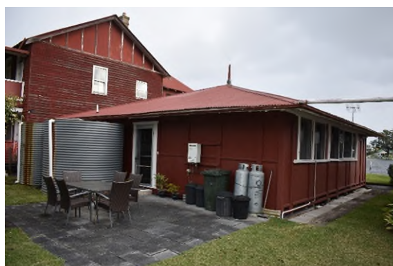
Figure 3.81 The rear (eastern) elevation of Building CM2.
