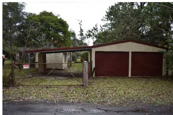
Figure 3.72 The outbuildings of Pamir (collectively referred to as Building P2).
