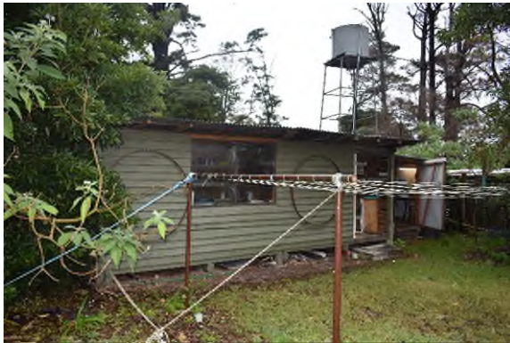
Figure 3.51 A laundry block, one of the outbuildings on the southern boundary of Block 10.
