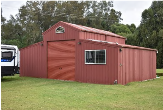
Figure 3.103 The fire depot, Building CM10.
