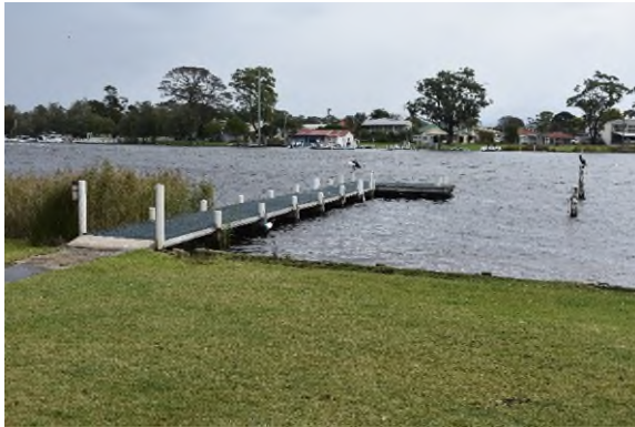
Figure 3.94 The jetty—structure CM6.
