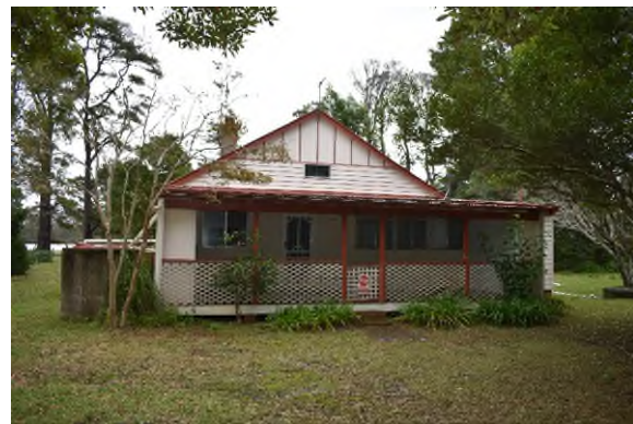
Figure 3.68 The eastern elevation of Pamir Cottage (Building P1), which fronts to the road.
