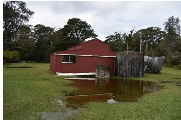
Figure 3.104 The rear of the fire depot shed, Building CM10.
