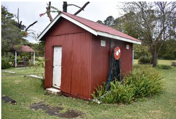
Figure 3.98 The western elevation of Building CM8, the site's pumphouse.
