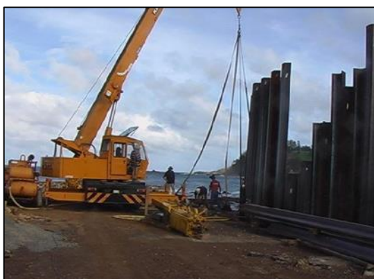
Figure 3-1 Installation of steel sheet piling.
