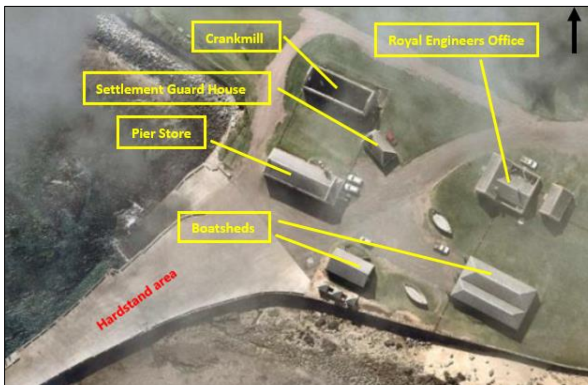
Figure 4-1 Land at Kingston Pier and nearby structures.
