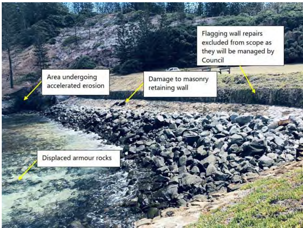
Figure 2-9 Location of rock revetment defects.
