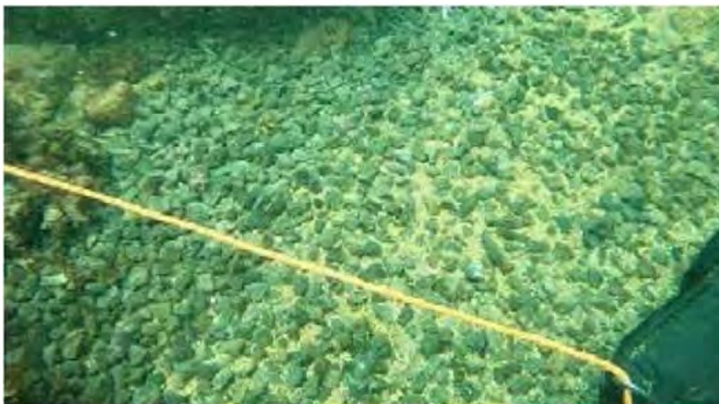
Figure 2-8 Loose gravel identified adjacent to sheet-pile wall.
