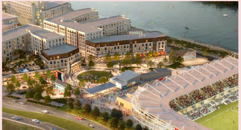
Figure 37. Billion dollar mixed-use development under construction adjacent to CPKC, the largest rail yard in North America, offering a mix of affordable housing and integrates with a streetcar extension.
