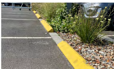
Figure 83. Wheelstops made from recycled plastic in Burwood, Victoria.
