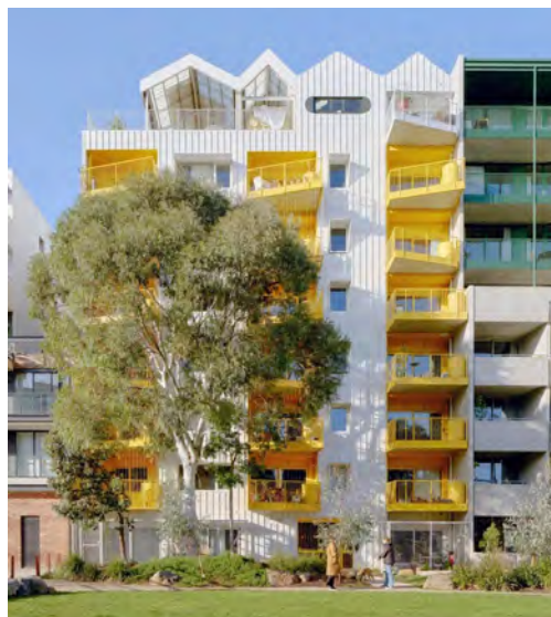
Figure 49. Parklife, Melbourne, VIC - Austin Maynard Architects
