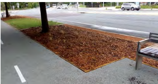
Figure 79. Porous paving on Barry Drive, Canberra.
