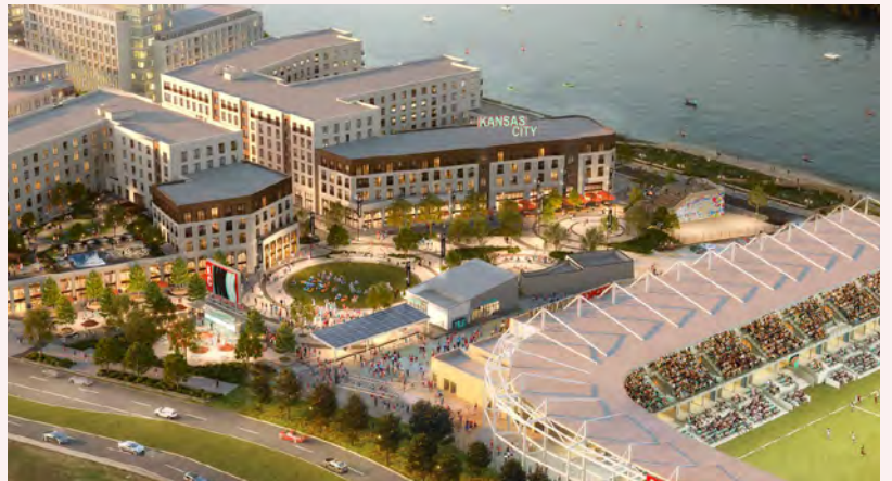
Figure 37. Billion dollar mixed-use development under construction adjacent to CPKC, the worlds first dedicated women's sports stadium in Kansas City, USA Project includes 10% affordable housing and integrates with a streetcar extension.
