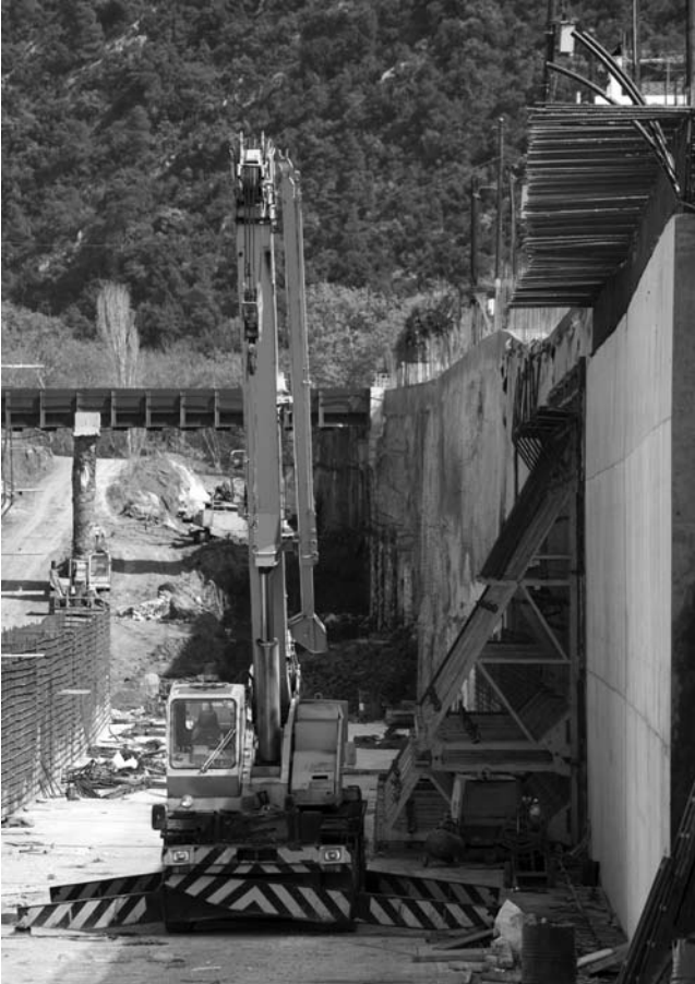
Road construction, Perth, Western Australia
